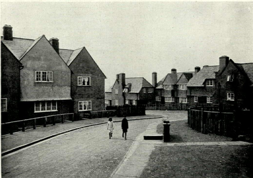
ENGLAND'S GOVERNMENTAL GARDEN VILLAGE. WELL HALL, WOOLWICH—VIEW OF WHINYATES ROAD.
