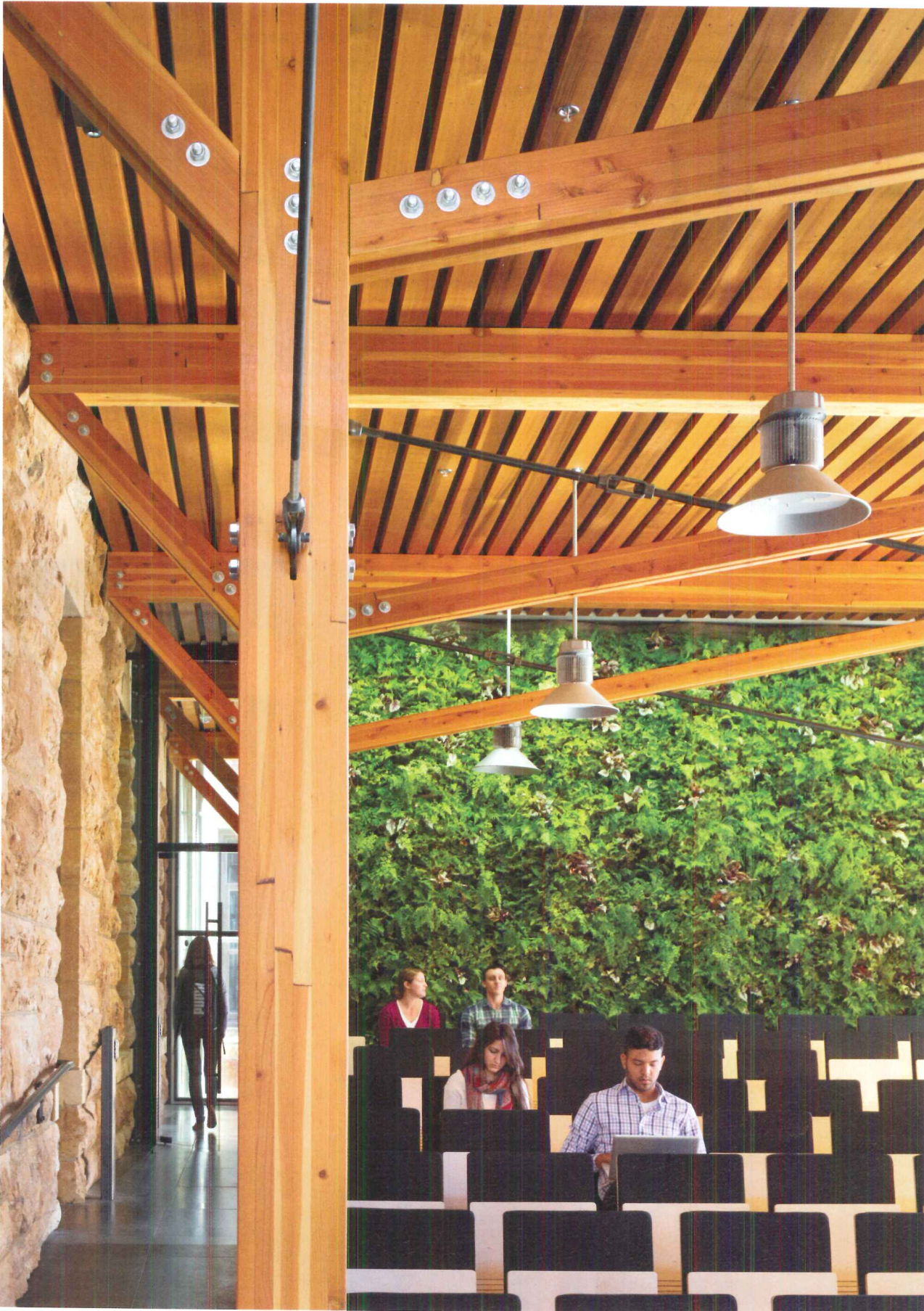
POST AND BEAM A heavy timber structure gives the new lecture hall (opposite) a turn-of-the-last-century warehouse feeling. The ferns and begonias growing on the hall's rear wall (left) are irrigated with stored rainwater.
