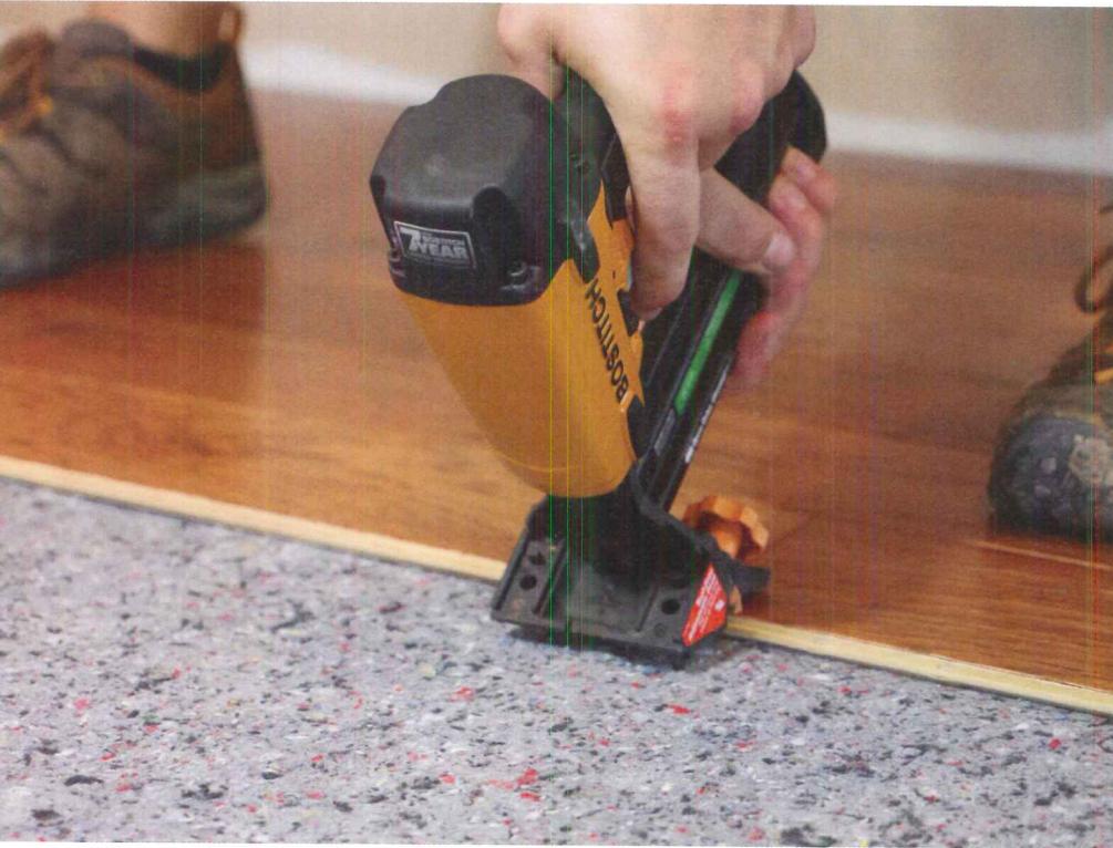
Underlayments of postindustrial and preconsumer recycled textile fibers are used to cushion the floor, dampen ambient sound, and absorb impact sound.
