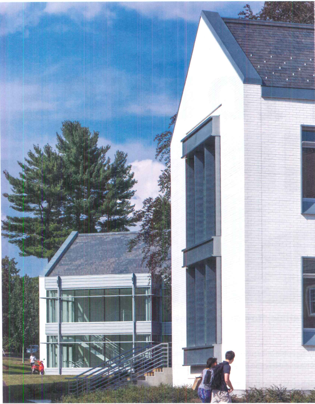
DECISIVE DETAILS Titanium zinc turns key elements of the building envelope—downspouts, gutters, and window frames—into expressive moments at the Lanphier Center for Mathematics and Computer Science at Choate Rosemary Hall (left, below, and bottom).
