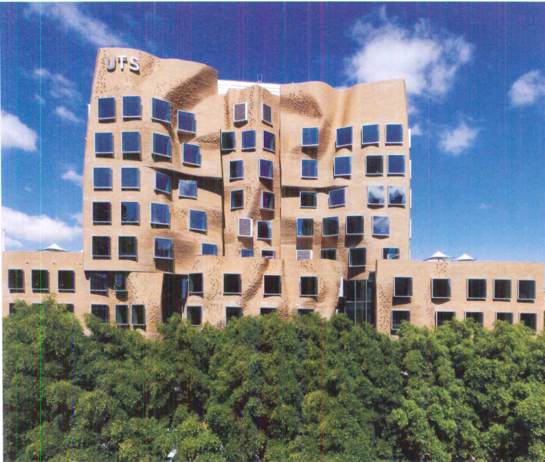
FROZEN FOLDS Despite its visual complexity, the facade of Gehry Partners' Chau Chak Wing (left and below) at the University of Technology Sydney relies on only five different types of bricks.
