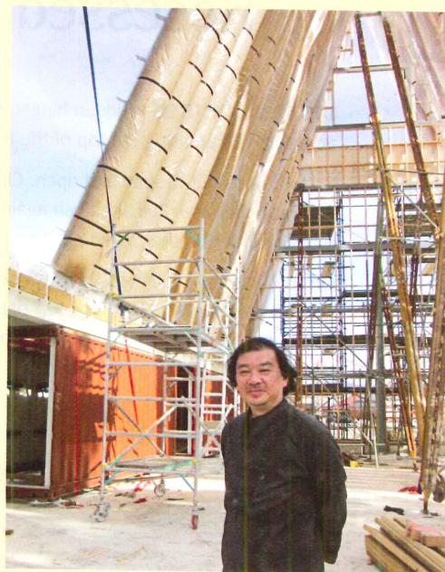
Shigeru Ban in front of his cardboard cathedral. The roof will rise up to 70 feet above the altar.
