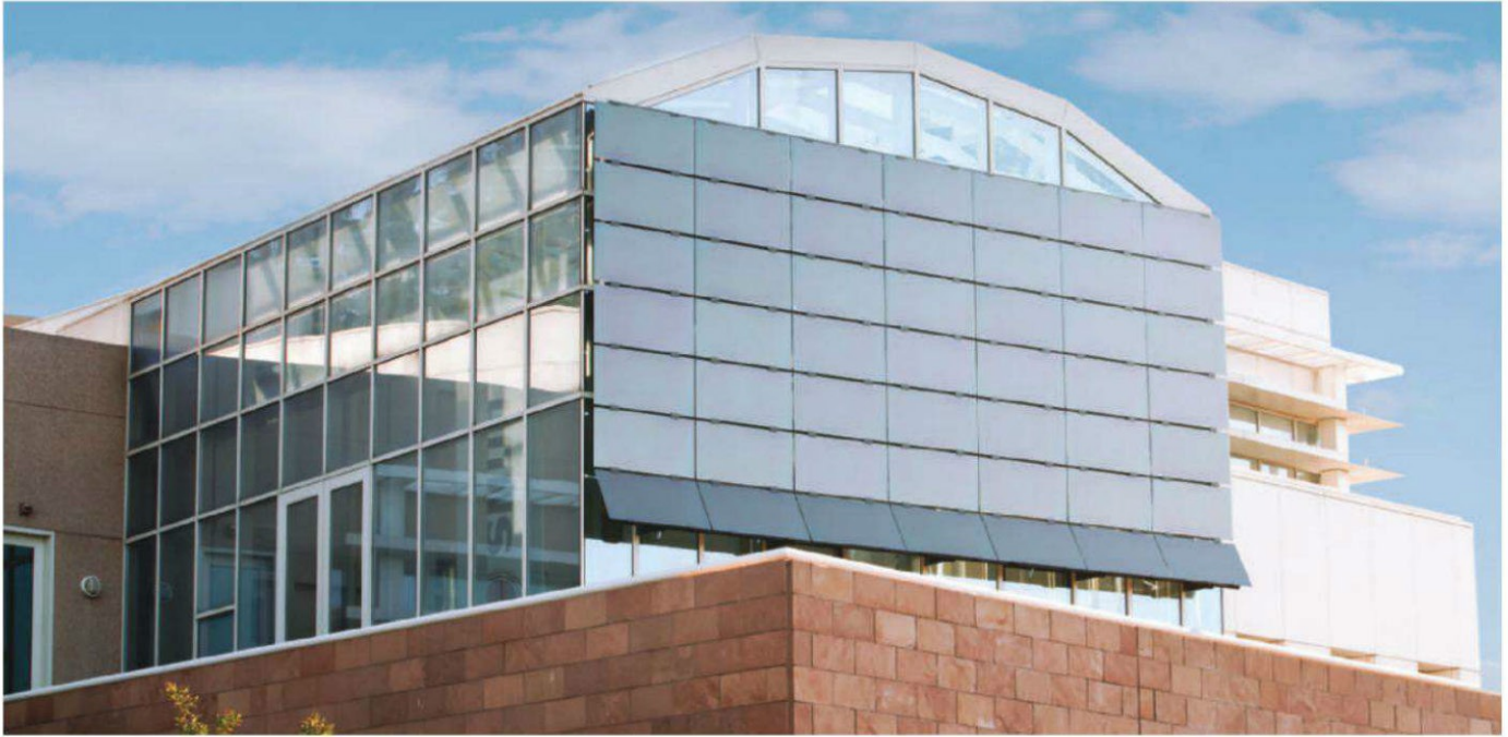
A UL-approved BIPV curtain-wall retrofit on the Sacramento Municipal Utility District (SMUD) Headquarters in Sacramento, California.
