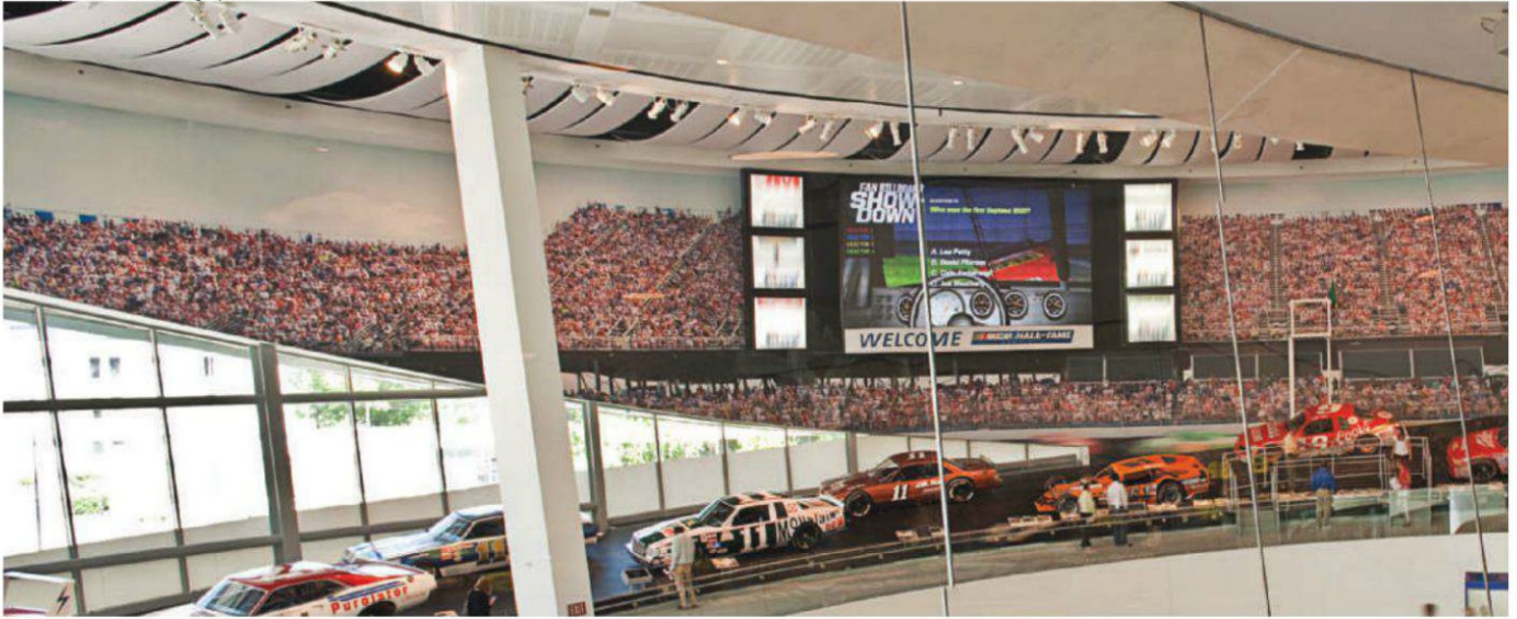
Charlotte, North Carolina's NASCAR Hall of Fame fan billboard, a 24-foot by 14-foot array of rear-projection digital display tiles, integrates high-impact visuals with brightness and clarity when viewed at any angle in a large space.
