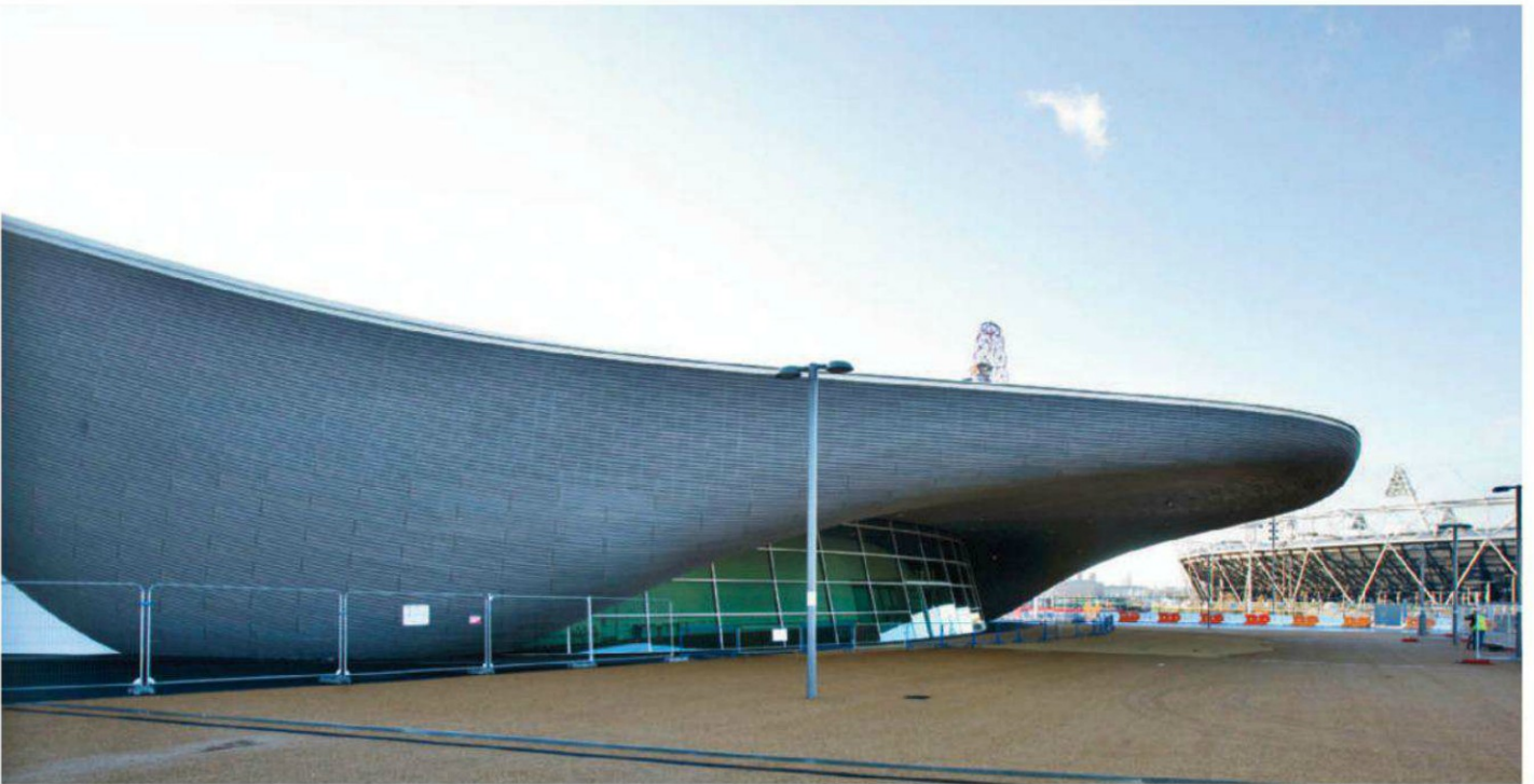
Aquatics Centre Zaha Hadid Architects
