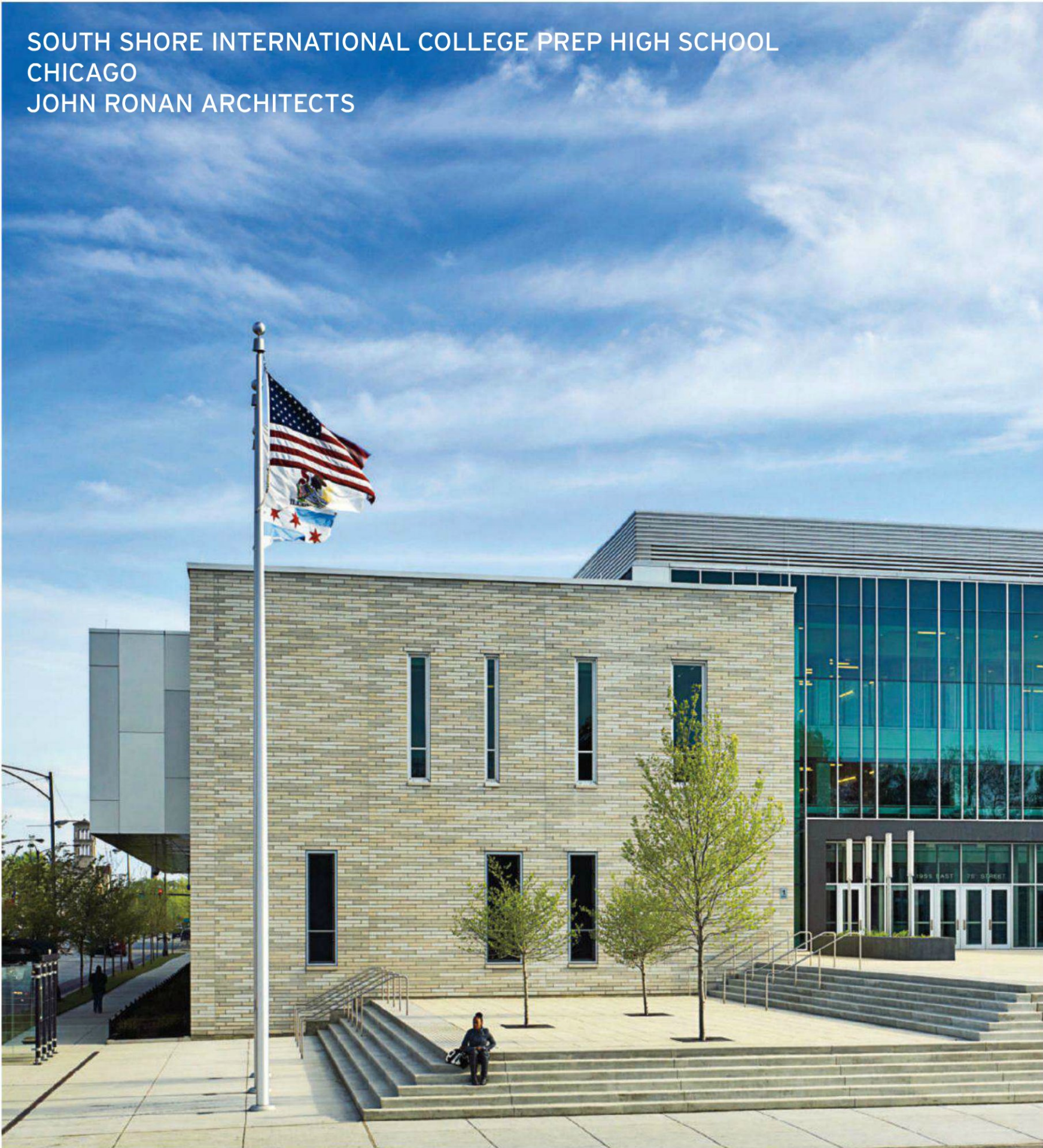
The high school's main entrance at the northeast corner is elevated on a plinth, which is intended to give the school a sense of importance as well as to provide sitting areas on the steps.
