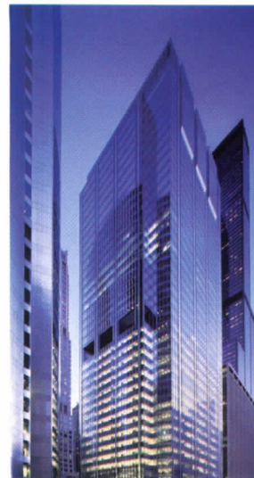
Custom Curtain Wall at 111 South Wacker designed by Goettsch Partners, custom-engineered by Oldcastle Glass®
