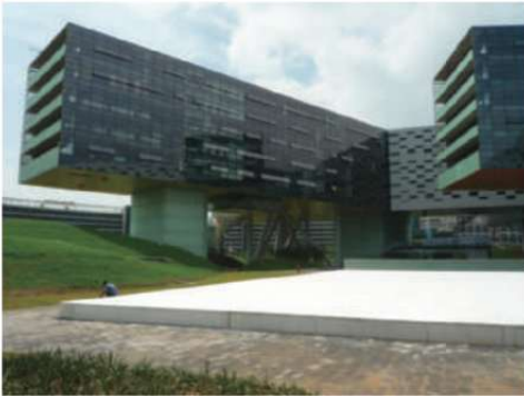
The cable-stay structure permits open facades.
