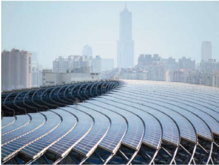
While shading the stadium's spectators, the aluminum-framed glazed roof panels – most of which are solar – harvest the sun's energy.
