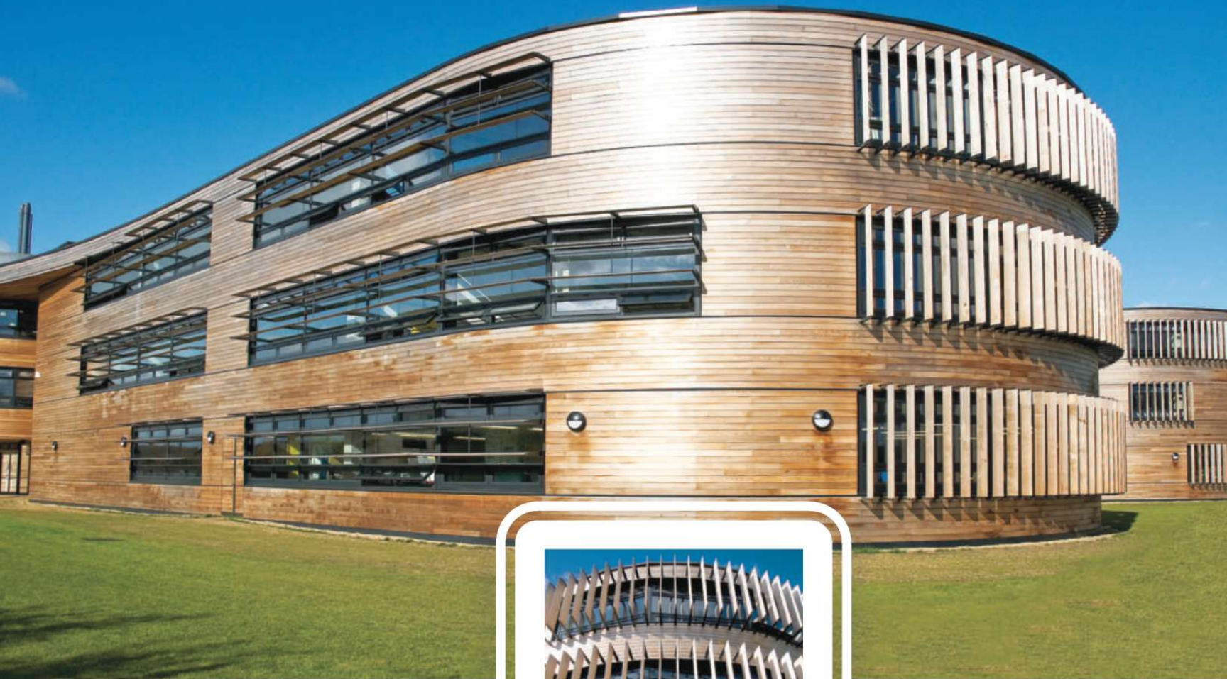
Langley Academy of Science, Berkshire, U.K. Architects: Foster + Partners Photo: Courtesy of Levolux Ltd.
