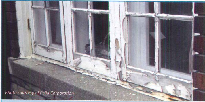
Window deterioration
