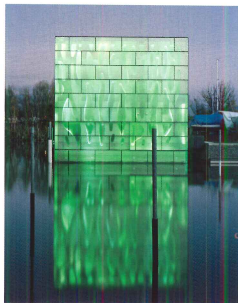
ABOVE: The reedlike concrete skeleton of Nordwesthaus is reflected through the exterior glazing onto the lake.
