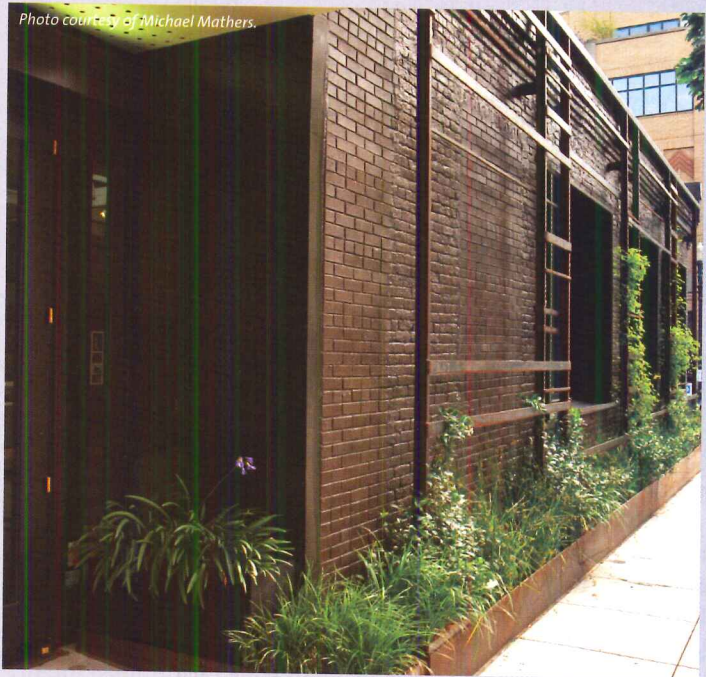
Photo courtesy of Michael Mathers. Through water-efficient fixtures and reused rainwater, the AIA reduced its annual potable water demand for toilets and urinals by 97 percent, plus provides for the Center's minimal irrigation needs.
