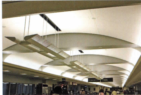
Claro finished panels in Ceilencio suspension
