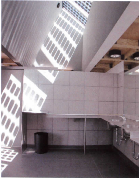
Aspen's Wagner Park Edge includes a glass-laminated photovoltaic installation as its sole power source (above and right).
