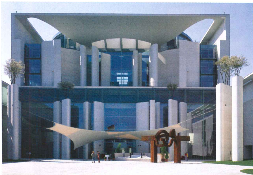
The Chancellery in Berlin, designed by Axel Schultes, stands as one part of a larger complex of buildings housing the executive branch of federal government, and brings to mind the work of Edward Durell Stone.
