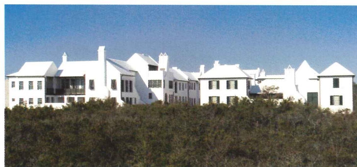
The houses of Audubon Village (top) are reinforced against wind; concrete stilts allow them to stand above potential flooding. Recently completed buildings in Alys Beach (above) mask their defenses in the style of new urbanism.
