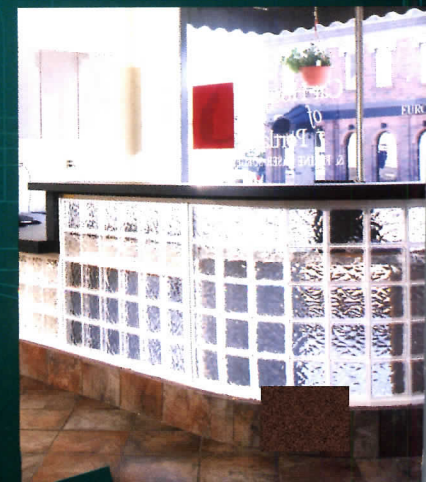
Aluminum mullions were used to connect these flat panels and radius walls together. A flat cap and mounting channel were used to mount the unit to the base and the walls. Flat caps were also used to connect the desktop to the top of the panel.
