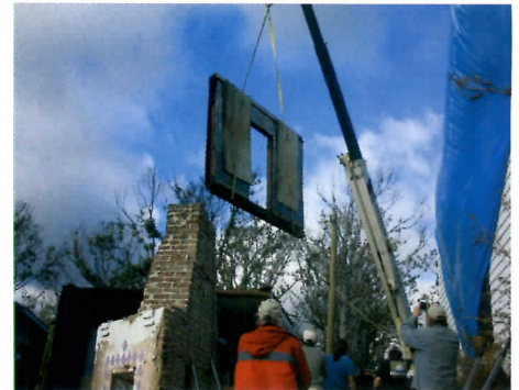
Workers dismantling the Hecker House.
