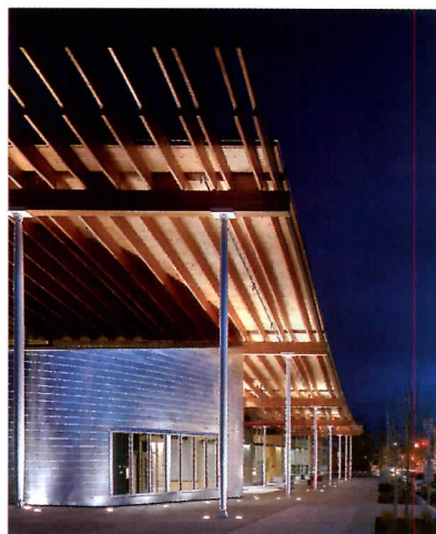
Ballard Library and Neighborhood Service Center, by Bohlin Cywinski Jackson.
