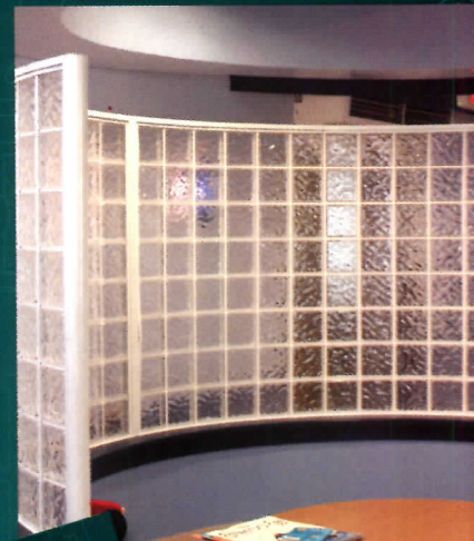
Round caps finished off the ends of this radius wall perfectly. Aluminum mullions were used to connect the three radius walls together, while a flat cap mounted the units to the top of the curved wall.
