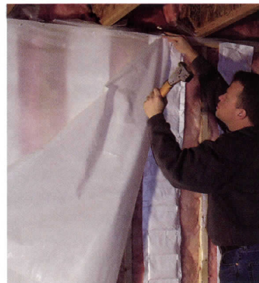
The strips are covered with vapor retarder.
