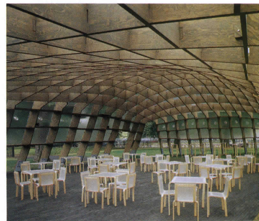
Interlocking timbers of 427 different lengths (above) create a column-free interior 56 feet wide (below).
