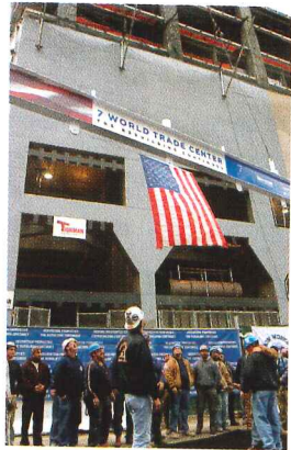
The final beam is lifted at 7 World Trade Center.
