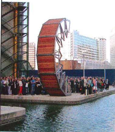
A pedestrian bridge in London makes waves by rolling out of the way (230).
