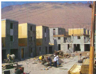
Elemental is building this low-income community in Iquique, Chile, for 100 families.
