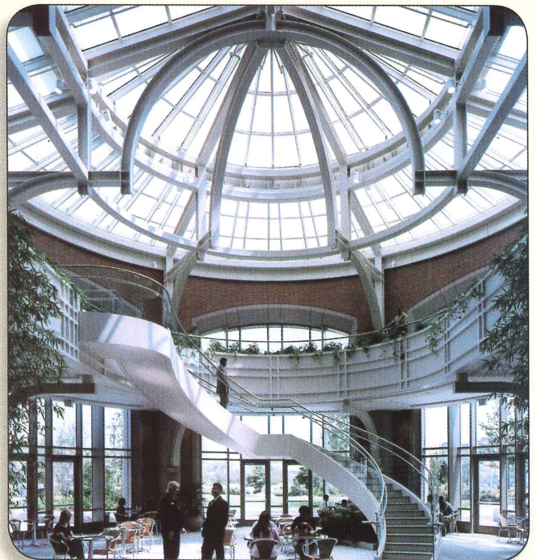
Photo: World Trade Center East, Boston, MA. Architect: Shepley Bulfinch Richardson & Abbot Architects Photo: Peter Vanderwarker. A/D FIREFILM® II on structural steel
