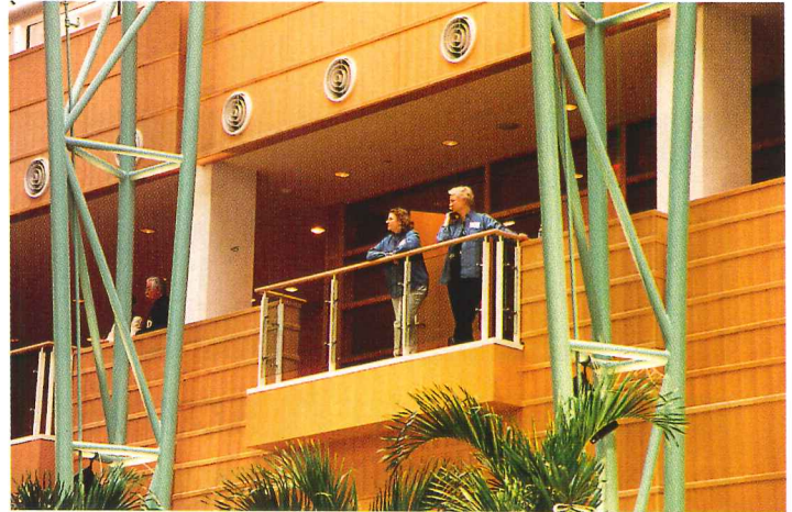
The atrium structure is separated from the theater wall by an acoustic joint.
