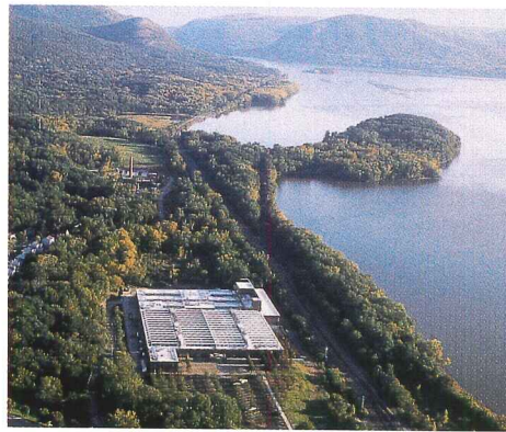
A Hudson River factory offered 292,000 square feet for exhibitions. Artist Richard Serra chose a former freight shed for his Torqued Ellipses (opposite).
