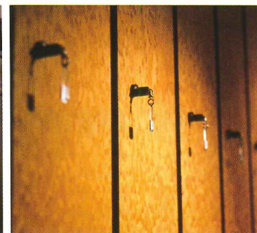
Decorative laminates allow architects to choose from an array of wood species that some consider an improvement on nature. From popular cherry and oak to lacewood, mahogany and teak, the designer can incorporate grain, color and finishes without the inconsistent flaws, knots and imperfections of wood veneers.
