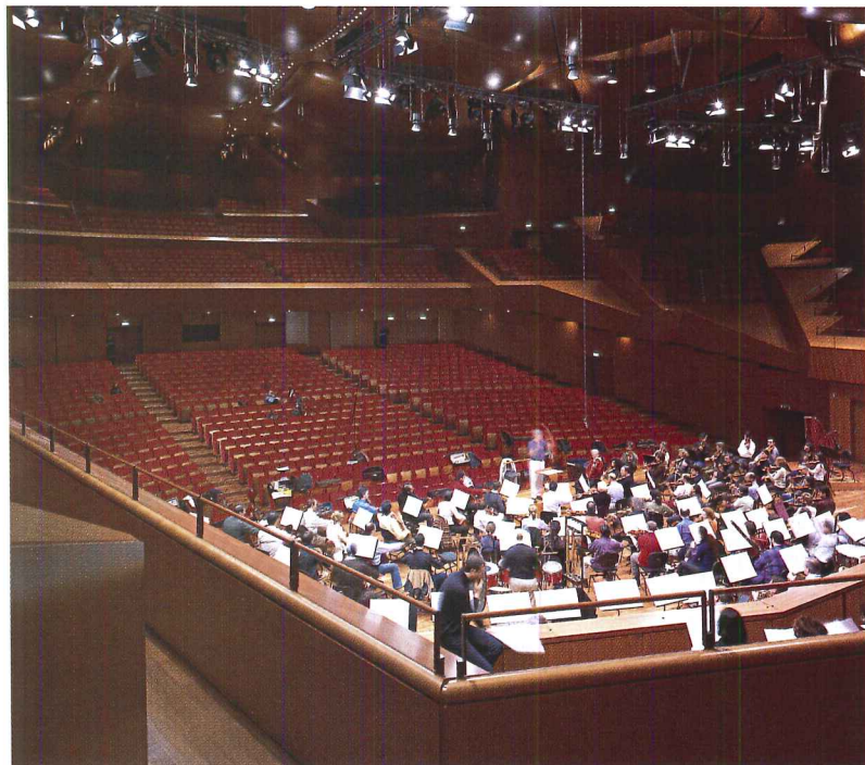
The two smaller concert halls (above and left) are highly flexible acoustically, with adjustable cherry ceiling and wall panels. But the most elaborate acoustic forms belong to the symphony hall (top), where 26 ceiling hulls are sized and shaped to disperse sound and resolve echoes.
