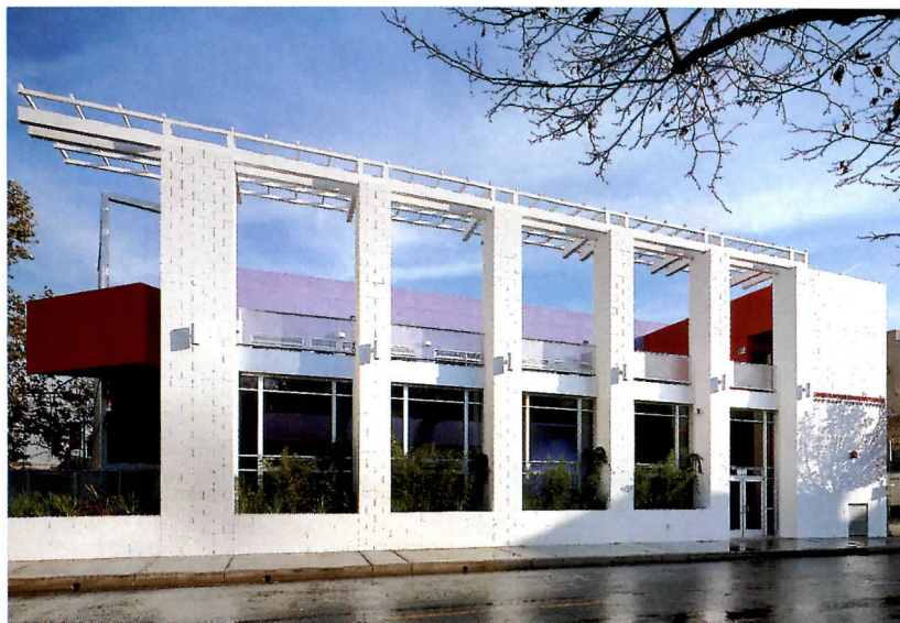
Designed by Lehrer Architects, the James M. Wood Community Center, in L.A.'s skid row, brings good design to a population that rarely has an opportunity to appreciate it.
