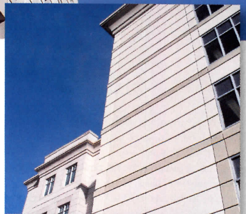
Dimension Series with Duracast matches an adjacent precast building (background).
