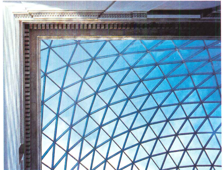
The glass-and-steel roof appears to float weightlessly over the Great Court. The grid is made of 3,312 unique glass triangles fritted to reduce solar gain.
