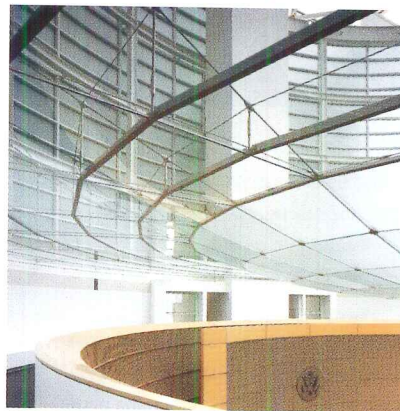
View from above the lens ceiling during construction (above). A visitor's view of the ceiling (below). Sprinkler pipe and cables were invisibly integrated (right).
