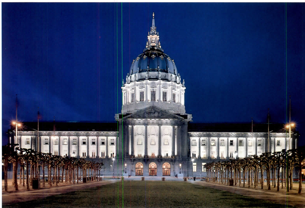
The largest rotunda in the United States glows in the night sky, with the help of long-beam metal-halide spots installed on the roof and dome base. Other metal-halide fixtures are hidden on ledges and cornices.
