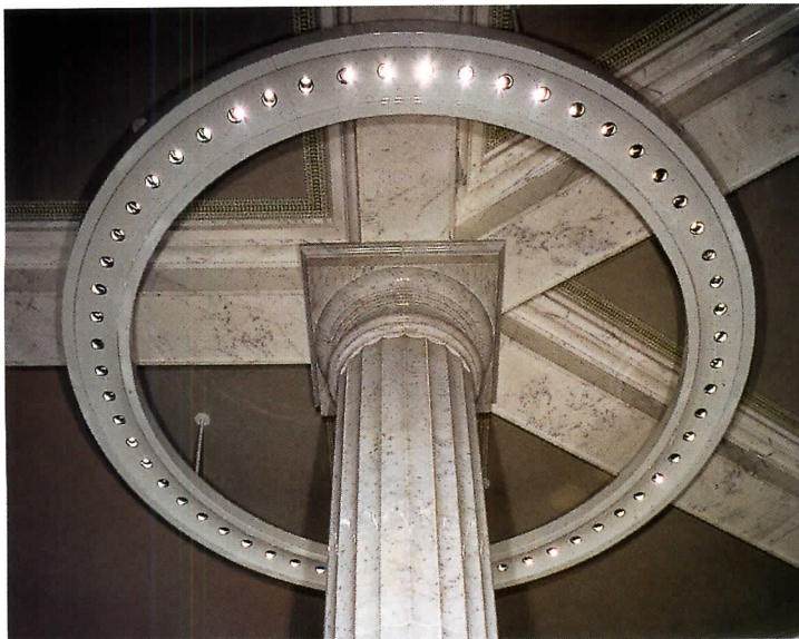
A new 14-foot-diameter ring made from fiberglass-and-resin composite houses 60 SOLUX lamps to light the Marquette Building's Tiffany mosaic.
