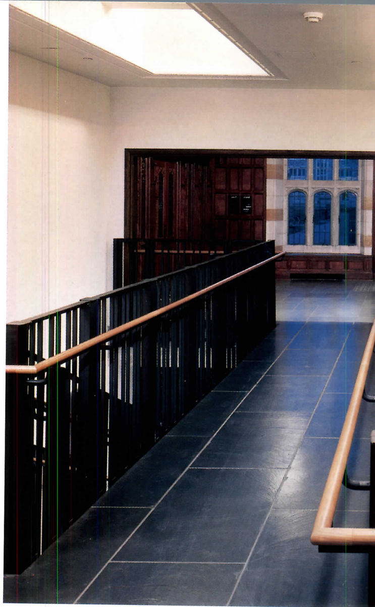
room (opposite, top right). Battens, holding insulation, screen stairs and chair storage. Wood panels reverse to dance-studio mirrors.
