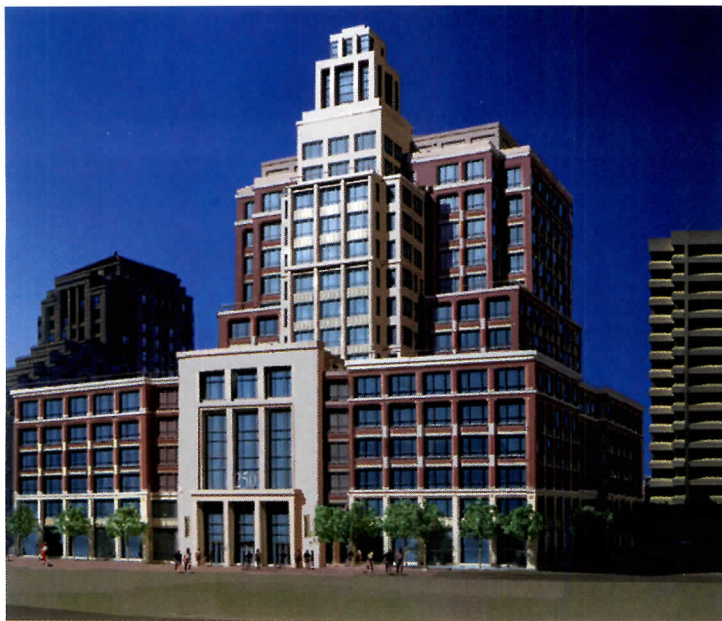
The Gap Embarcadero (above), by Robert A. M. Stern Architects and Gensler, includes slotted-web connections and a seismic core (below).
