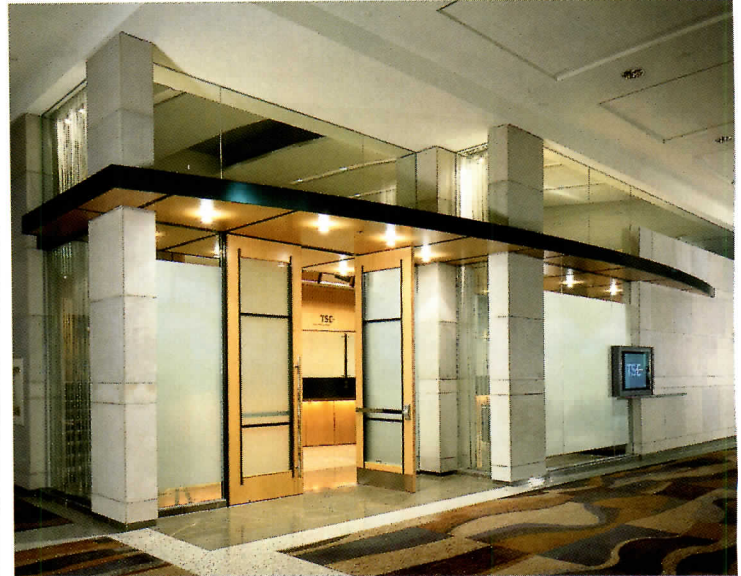
The new entrance to the conference center of the Toronto Stock Exchange provides a formal welcome to visitors arriving through an adjacent retail mall. A canopy wrapped in beech veneer is fitted with MR16s that add a bit of sparkle.
