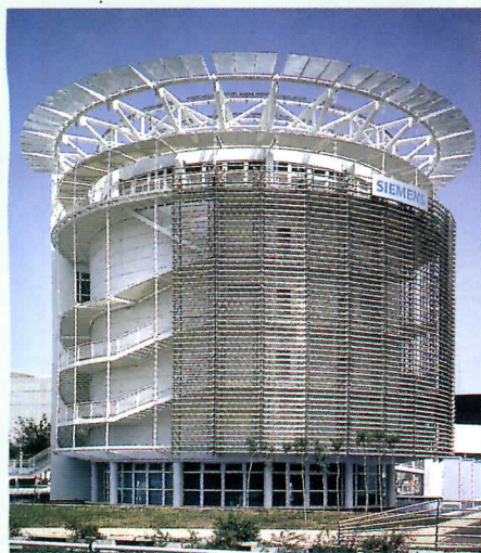
The Siemens Pavilion (above), built for Sevilla, Spain's 1992 exposition, uses a seasonally adjusted prismatic sunscreen to protect the building from the sun. The 3M Corporation's Austin Center uses a mirror system (right, top, and middle) and the company's prismatic film to light the building's atrium (bottom right).
