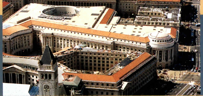
Looking west over the Rios Building to the new Reagan Building.
