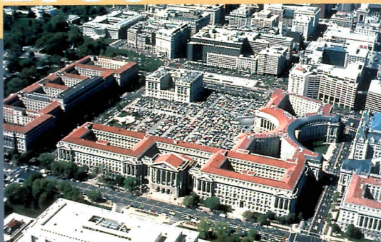
Site of the Reagan Building when used as a parking lot.
