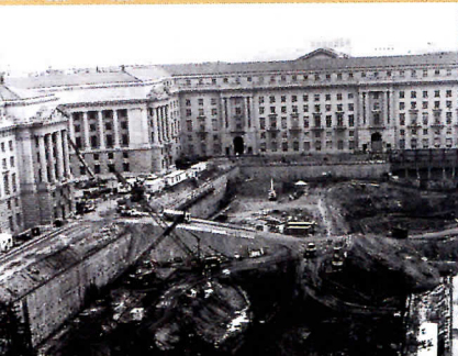
Preparing the site for construction.
