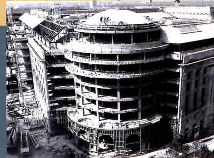
Pennsylvania Avenue rotunda being built.
