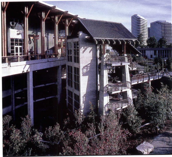
Project: REI Flagship Store Seattle, Washington Client: Recreational Equipment, Inc. Building Type: Retail Award Category: Private sector, over $25 million Key Players: REI—Wally Smith, Jerry Chevassus; Mithun Partners (architect)—Bert Gregory, AIA, Thomas Emrich, AIA, Robert Deering, AIA
