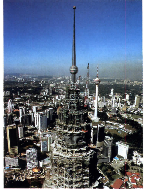
At the Petronas towers (above), high-grade concrete and self-climbing forms helped erect the world's tallest buildings faster.
