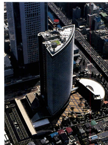
(above right). The office tower’s curtain wall (section above) is shaded by projecting metal fins (four per floor) on the outside and blinds on the inside. A perimeter air-handling system lets the curtain wall breathe by conditioning air as it comes in.
