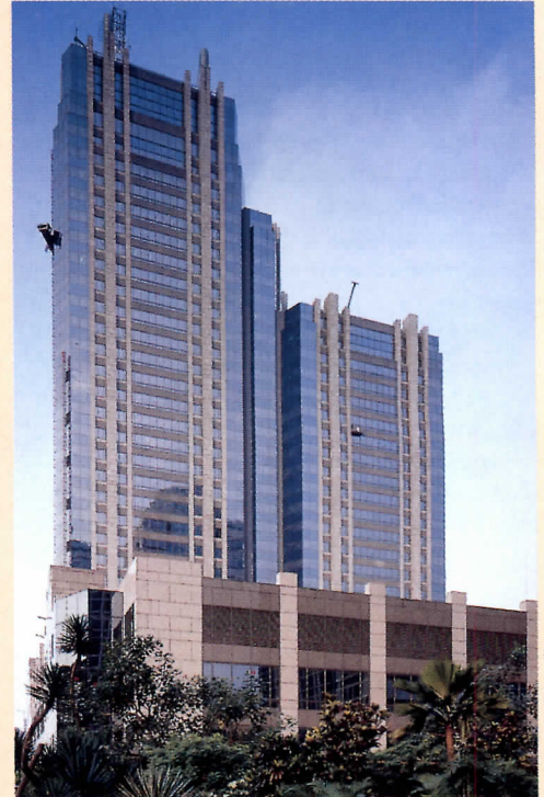
Jakarta Stock Exchange, by Brennan Beer Gorman, rises in a new business district.
