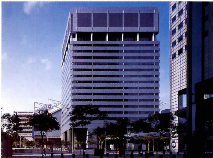
At 570 feet by 475 feet, the convention center's external space-frame roof (opposite and drawings above) is one of the largest in the world. The 18-story office tower (left) has large (28,000-sq.-ft.) floor plates to attract international tenants.
