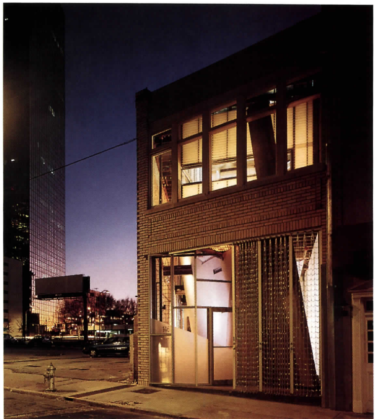
Located in a mixed-use neighborhood, the 3,000-sq-ft building retains an industrial esthetic. Its simple masonry shell (top) serves as a foil for a dynamic interior. An angled glass wall recessed within the building's mass creates a covered entry space that can be closed from the street by a chain-metal curtain (above). The main staircase is assembled from yellow-pine 2x10s and 2x12s (opposite).
