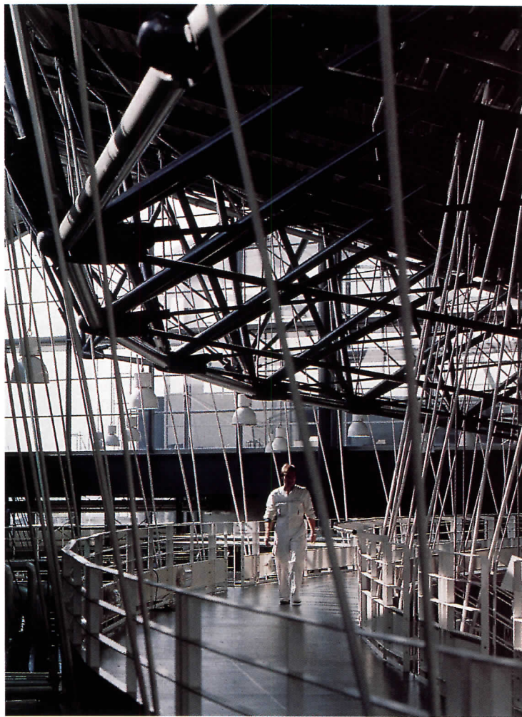
The architects and engineers used structures and materials to make the factory's interior as light and open as possible. For example, the curtain wall at the building's gable ends works with the bulging form of the roof to bring sunlight into the production area (left and above left). A second-story walkway is suspended from the roof and overlooks the manufacturing floor (above right).
