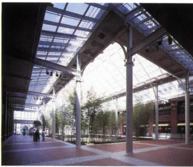
1990: Harborside, Jersey City, New Jersey
