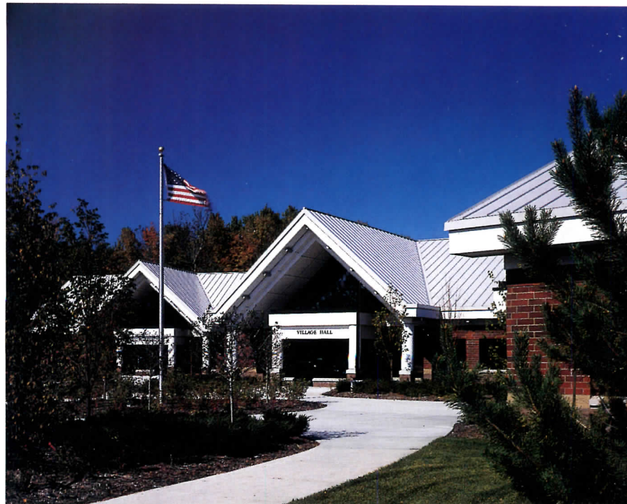
Orono City Hall Architect: Boarman Kroos Phister Rudin & Assoc. Roofing Contractor: Vohnoutka Roofing & Sheet Metal Co., Inc. Color: Sandstone
