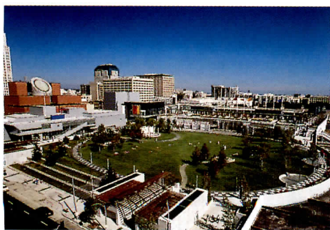
In front of the Botta-designed museum is MGA Partners' $23-million Yerba Buena Esplanade, which links Center for the Arts buildings by James Stewart Polshek (right in photo) and Fumihiko Maki (left).
