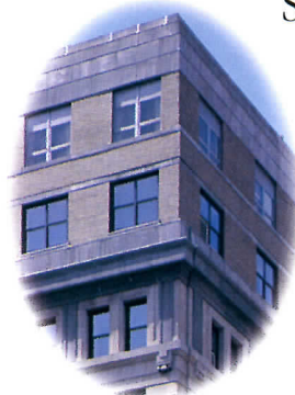
Hotel du Pont; Wilmington, DE: Clear Float Glass outboard and Energy Advantage Low-E Glass inboard; renovation project.
