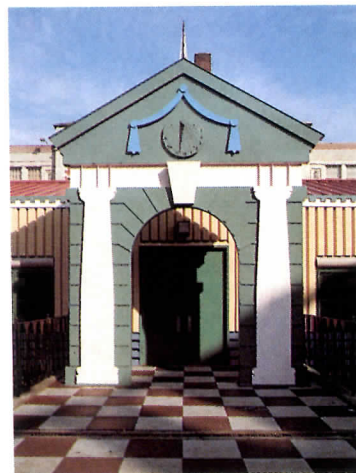
Using the same kind of pre-engineered construction that had previously resulted in unadorned metal sheds, architects Weintraub & di Domenico designed a series of lively school annexes for New York City (above and right). The rigid-frame, metal-skin structures provide fanciful elevations for classes to pose in front of and windows set at a child's height.
