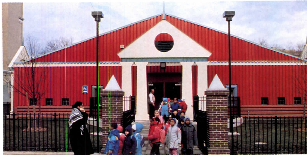
Using the same kind of pre-engineered construction that had previously resulted in unadorned metal sheds, architects Weintraub & di Domenico designed a series of lively school annexes for New York City (above and right). The rigid-frame, metal-skin structures provide fanciful elevations for classes to pose in front of and windows set at a child's height.
