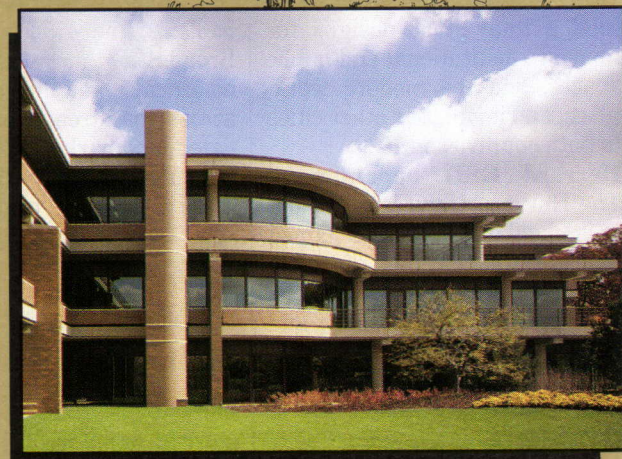
Architect: Lohan Associates Roofing Contractor: Olsson Roofing Company Carlisle Manufacturer's Representative: Cambric Corporation
