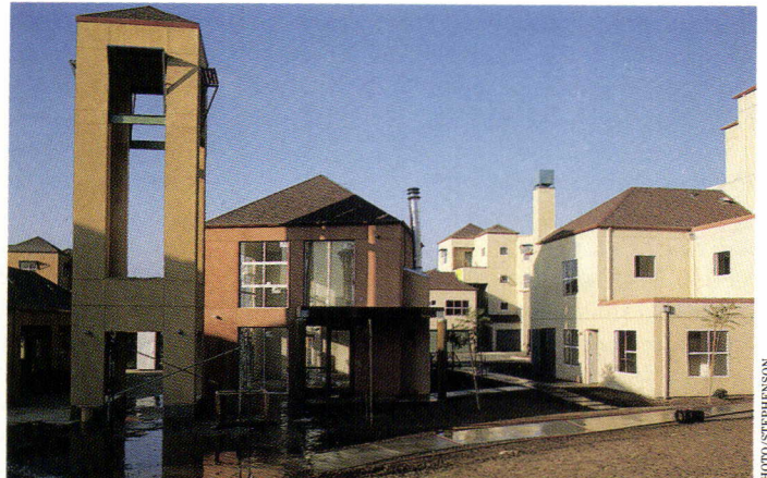
Fisher Friedman Associates designed a student housing complex to give it a villagelike character.
