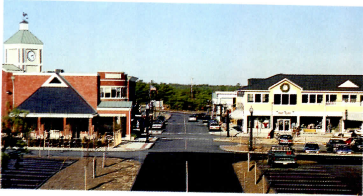
Although Fields Point Limited elected to incorporate its 1962 New Seabury Shopping Center (top) into Mashpee Commons, using part of the earlier complex to define the southern edge of Market Street
