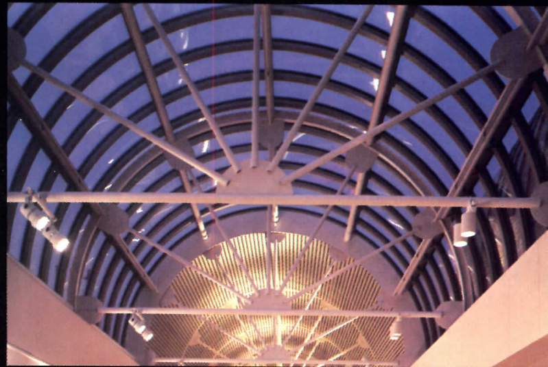
With a proprietary UV-resistant surface, LEXAN XL sheet is ideal for barrel vaults, covered walkways and skylights.
