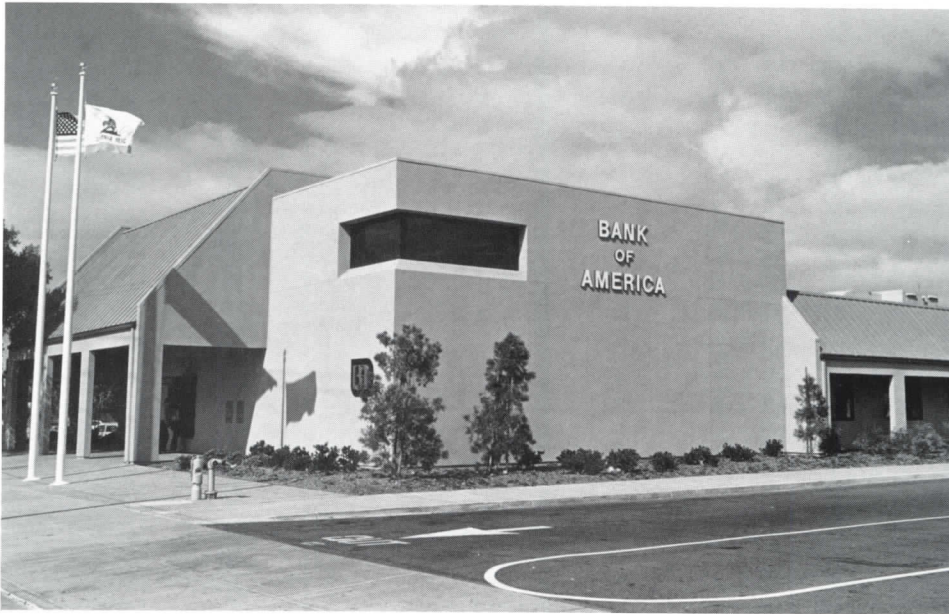
Conventional exterior of Bank of America's Livermore branch uses novel cooling system based on ice bank storage.
