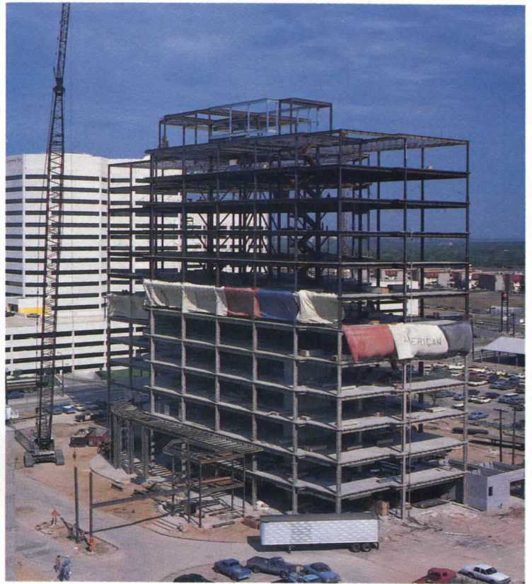
Vulcraft deliveries eliminated "lay down space" worries
