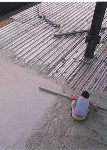
Composite deck simplifies construction
