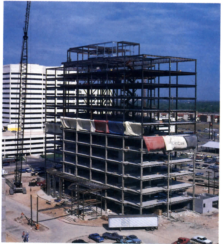
Vulcraft deliveries eliminated "lay down space" worries
