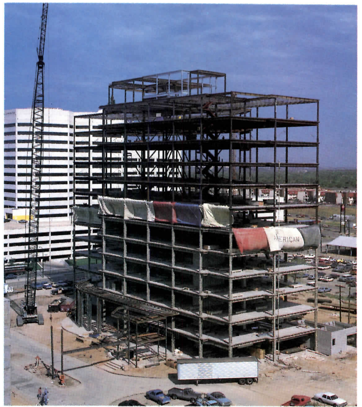
Vulcraft deliveries eliminated "lay down space" worries
