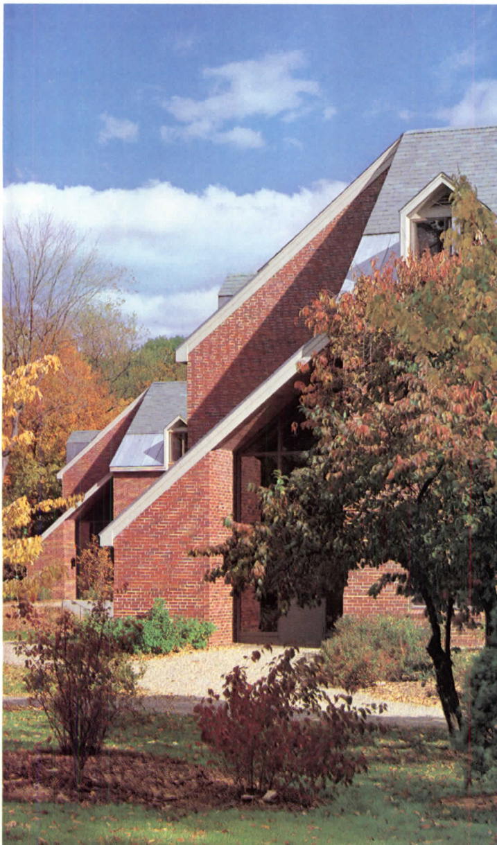
Principal entrances to both dormitories are tucked into the northwest corners and sheltered by a dropped pitched roof that replaces the expected hip at the right-angle intersection of the gables. Within, a triangular stairwell gives access to student room floors.
