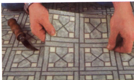
A Premier Sundial Solarian patch becomes a permanent part of the overall floor.
