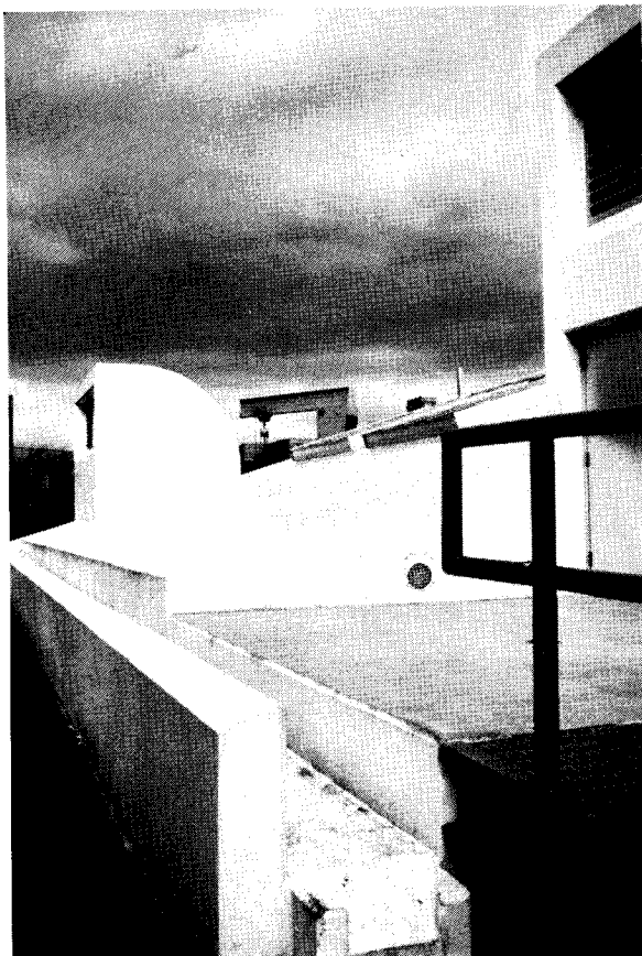
Sewage Pumping Station/Ramsey Dabby Photo
