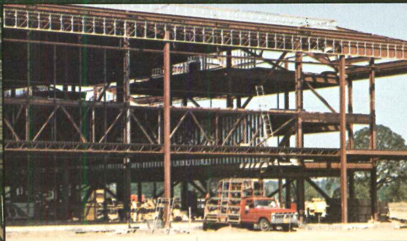
The versatility of designing with Vulcraft steel joists and joist girders helps meet complex design requirements like this unusual eight foot interstitial floor space.
