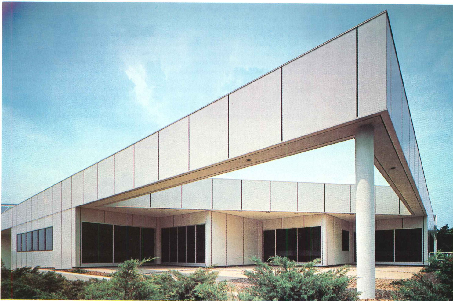
Project: Coastal Industries Office Building, Bath, Ohio Architect: Perkins & Will, Washington, D.C. Curtain Wall Erector: Handcraft Metals Corp., Cleveland, Ohio
