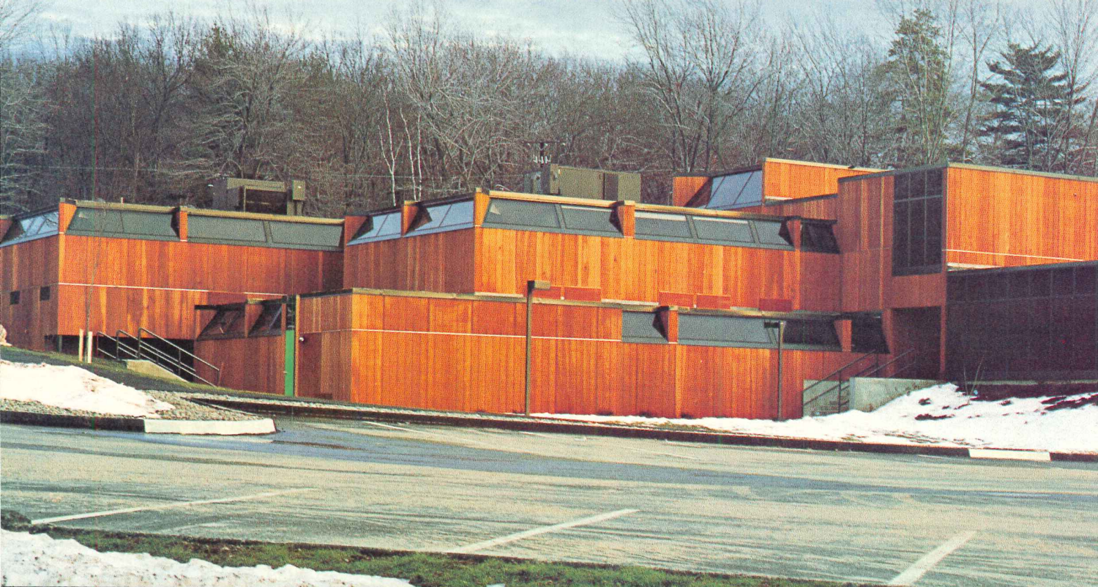
Medical Center—Andover, Massachusetts • Architects: Drummey Rosane Anderson, Inc.
