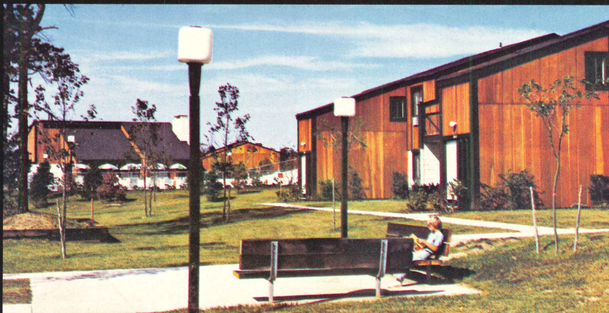
Nob Hill Condominiums—Hauppauge, New York • Arch.: John A. Jacobsen and Associates • Sponsor & Builder: The Campagna Development Corporation
