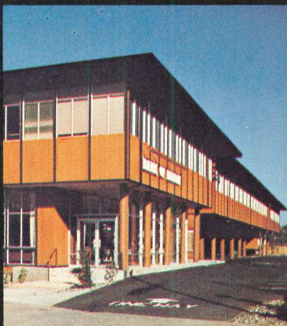
Office Building—Sausalito, California Arch.: Wurster, Bernardi and Emmons, Inc., AIA Structural Engineer: W. B. Clausen
