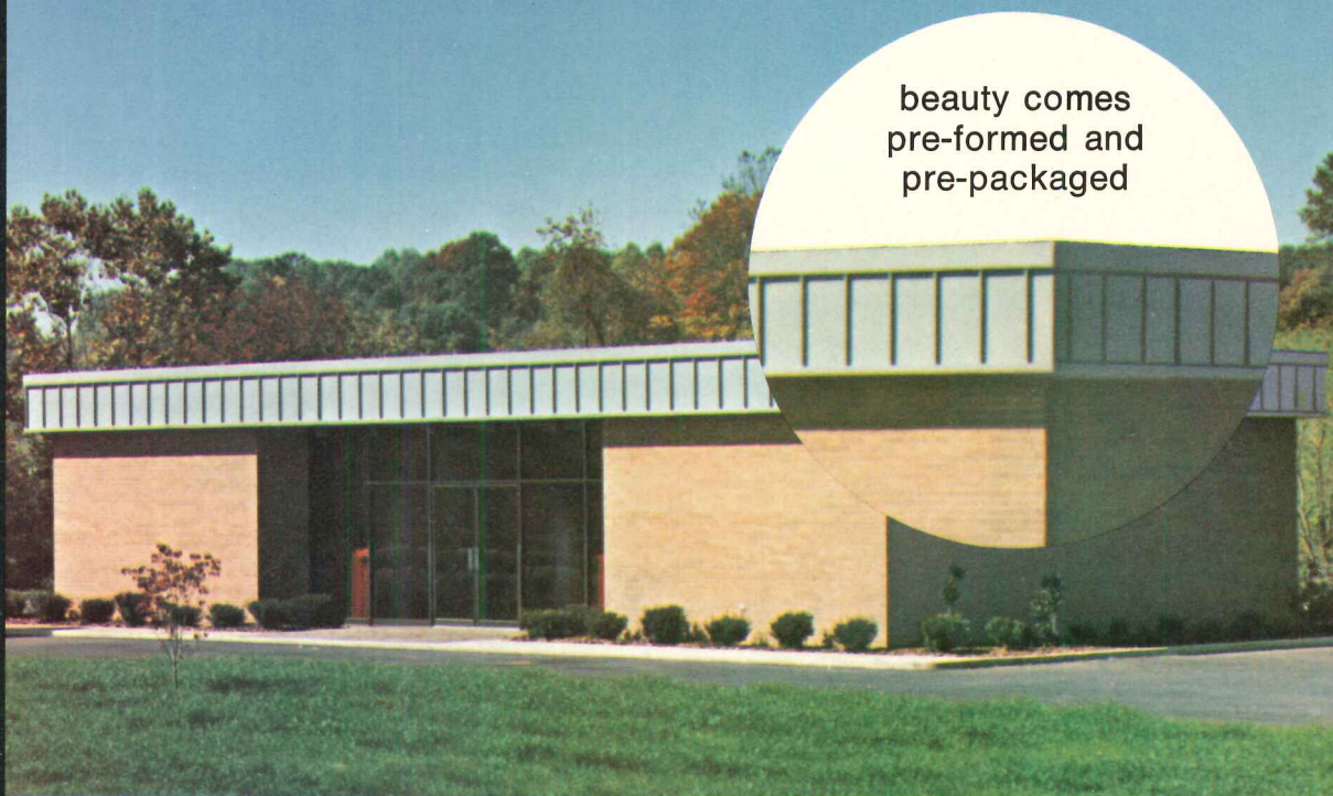
Greene County Bank, Greenville, Tenn., Architect: Boyd & Arthur, Roofer: Hicks Sheet Metal Co.
