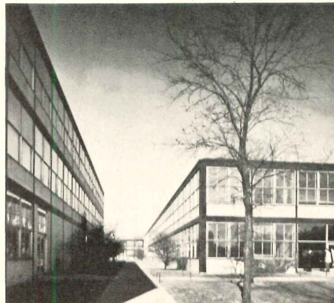
Illinois Institute of Technology, by Mies van der Rohe (1940-72)
