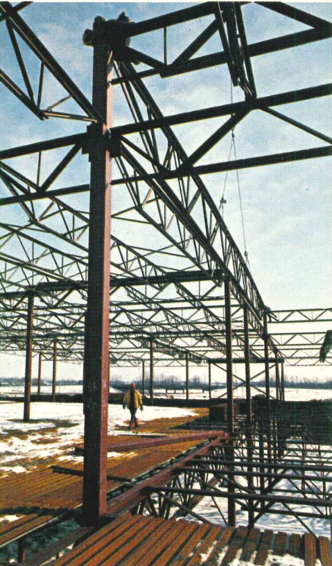
Wide spacing of deep steel joists (8" in floors and 7'6" in roofs) resulted in stiffer floor system and saving in the cost of joists.
