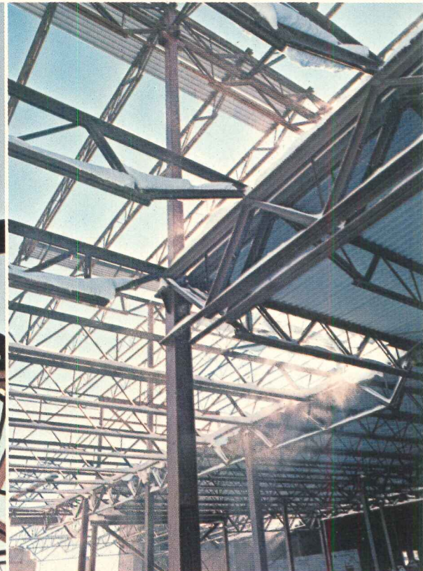
Joist girder design flexibility provided for a wide range of load support, from normal roof loads to heavy mechanical equipment loads.
