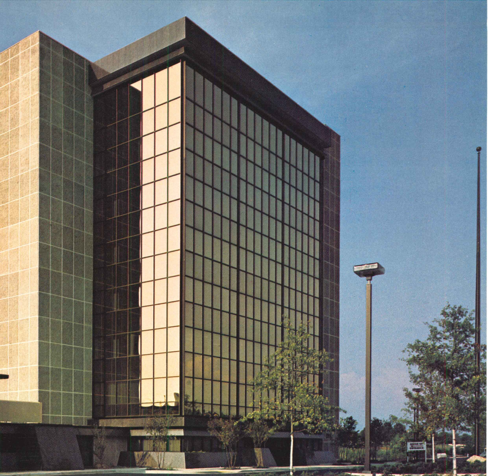
HOME FEDERAL SAVINGS & LOAN ASSOCIATION BUILDING Johnson City, Tennessee
