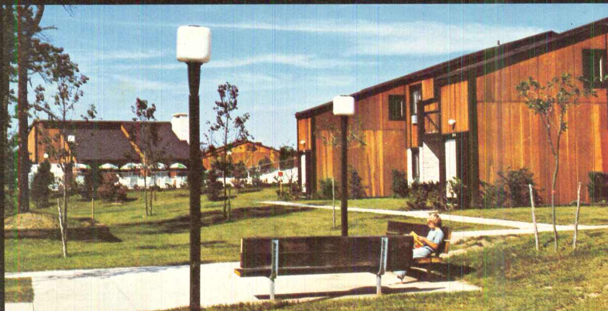
Nob Hill Condominiums—Hauppauge, New York • Arch.: John A. Jacobsen and Associates • Sponsor & Builder: The Campagna Development Corporation
