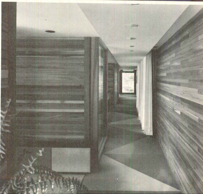
The principal finish materials are cedar siding, drywall, carpet, travertine marble, ceramic tile and bronze glass, which are used in generous amounts. The detailing of these materials, as in the carpet (photo left), is designed to reinforce the triangular vocabulary of the house.
