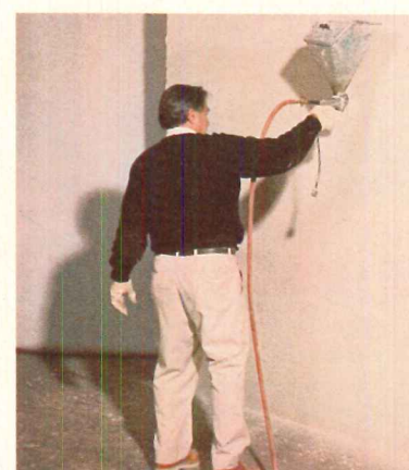
attractive, textured finish coat is sprayed over the prime coat. Both prime and finish coats can be troweled or sprayed. The result is superior insulation and an attractive finish shown at the right.
