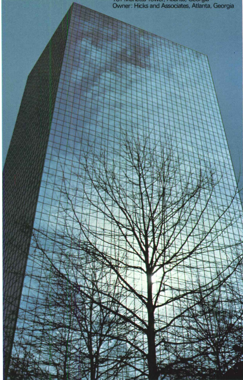
101 Marietta Tower, Atlanta, Georgia Owner: Hicks and Associates, Atlanta, Georgia
