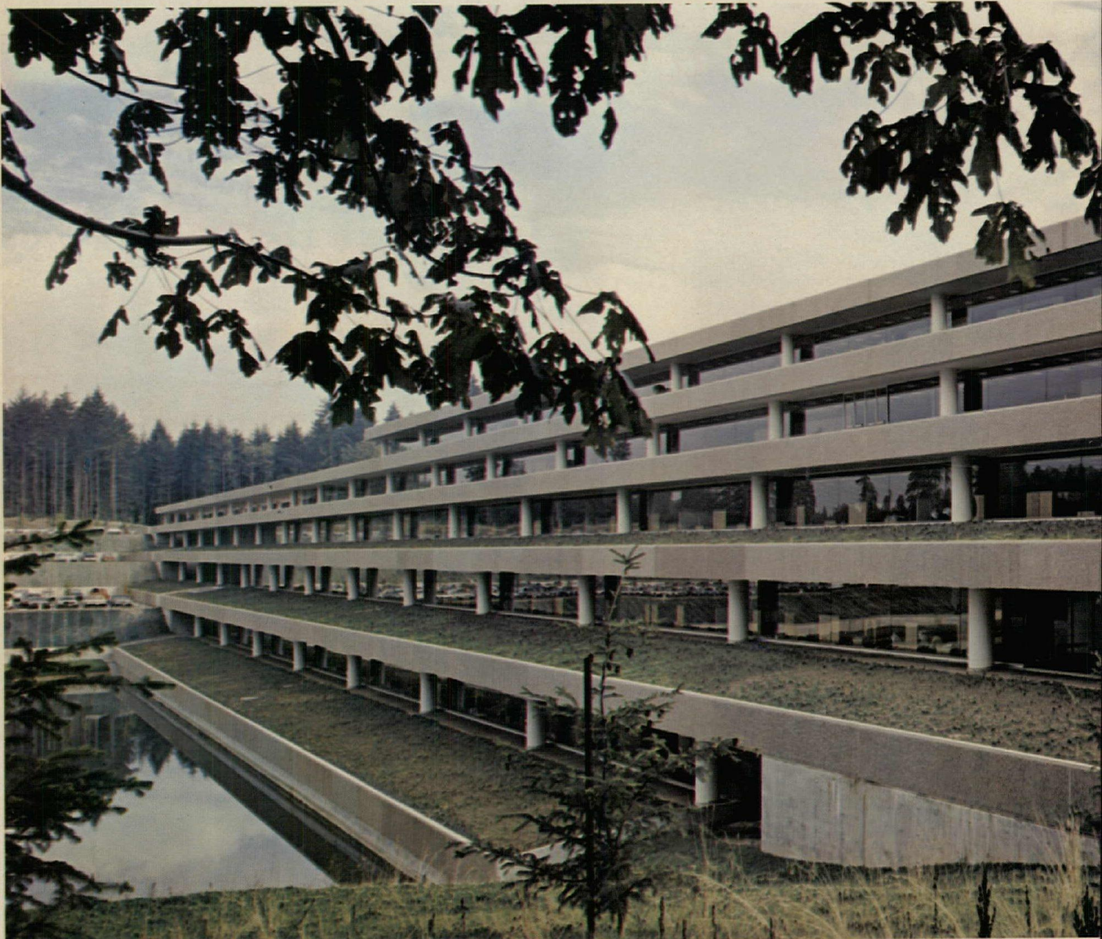
Owner: Weyerhaeuser Company, Tacoma, Washington. Architects: Skidmore, Owings & Merrill, San Francisco, California. Building Contractor: Swinerton & Walberg, San Francisco, California. Glazing Contractor: Cobblestick-Kibbe Glass Co., Oakland, California.
