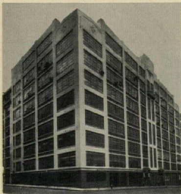
Nine-story, 180,000 sq. ft. building, 160 Jay Street, Brooklyn, N.Y. Building Owner: Cama Company, Brooklyn, N.Y. IRON FIREMAN Dealer: Oil Burner Utility Company, Inc., Long Island City, N.Y.
