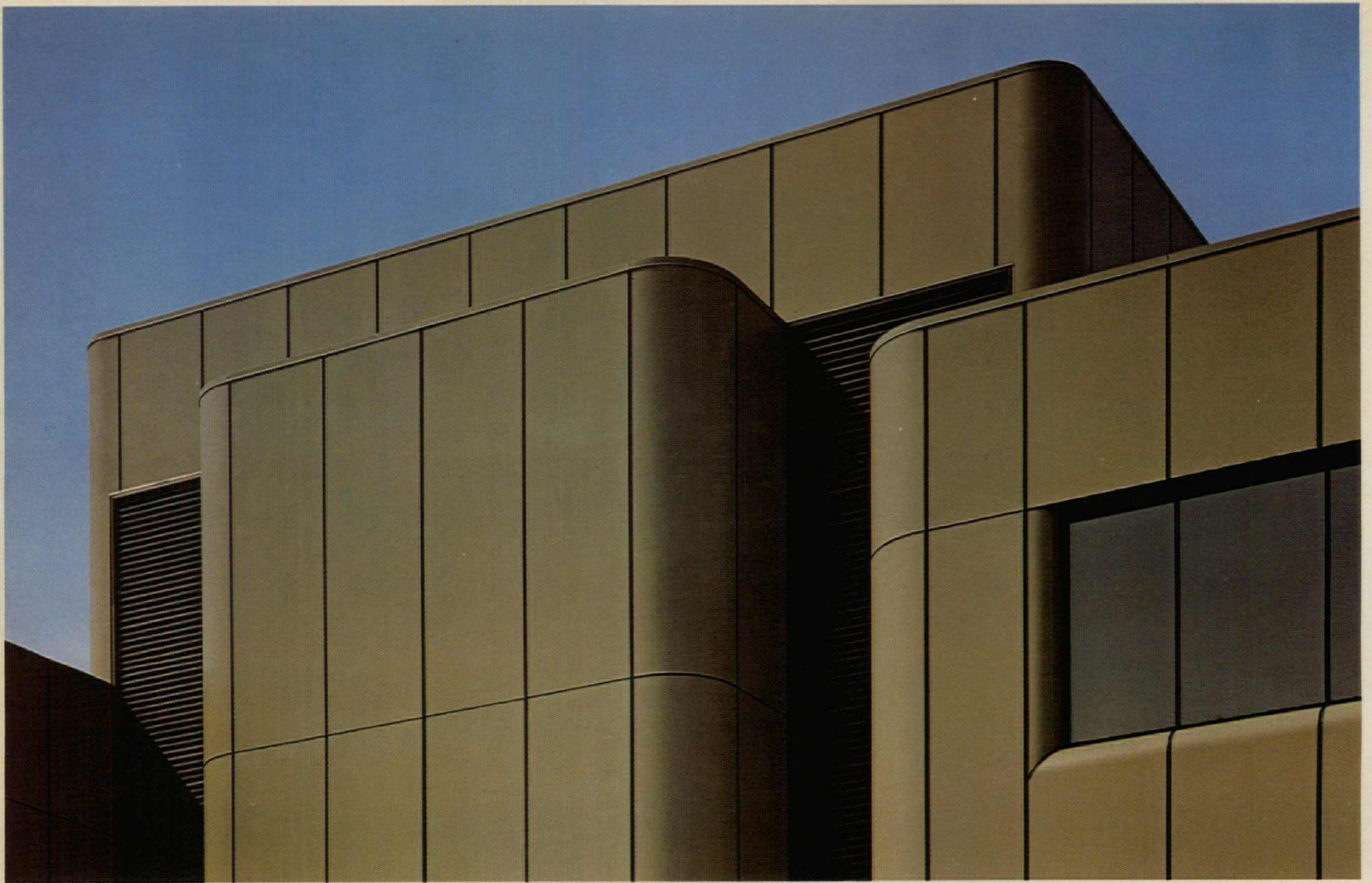
Project: Keen College Academic Building, Union, N. J. Architect: Robert Hillier, Princeton, N. J. Curtain Wall Erector: Whelan Mfg. Co., Trenton, N. J.
