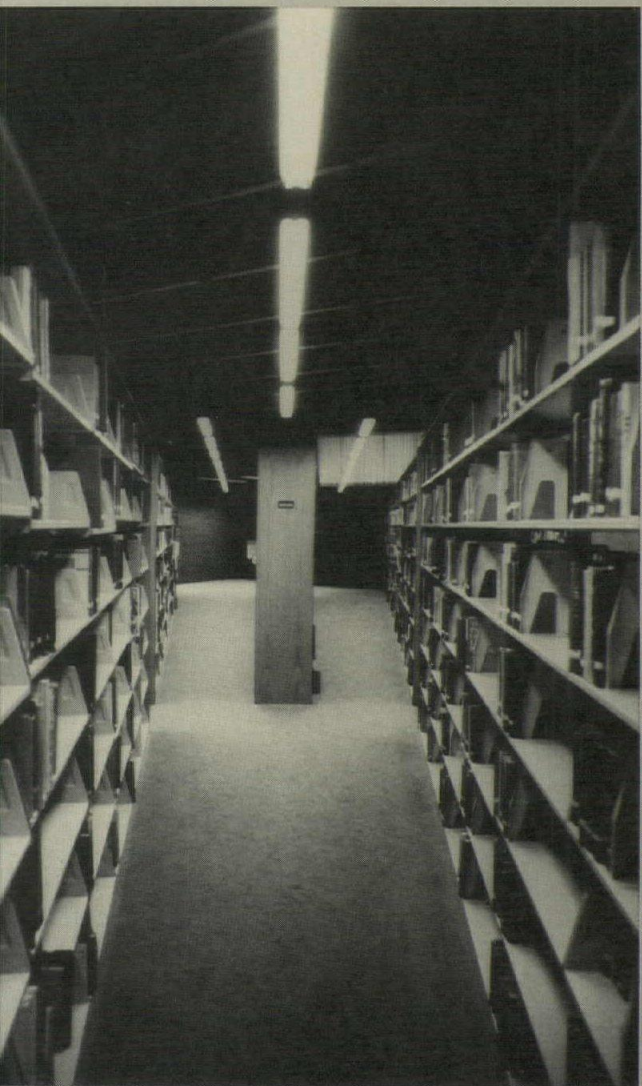
Electrified track in the ceiling of the Pekin library will allow luminaires to be easily moved to accommodate additions to the book stacks, to allow exhibit lighting to be changed in the lobby, and to permit rearrangement of furniture such as carrels and tables.
