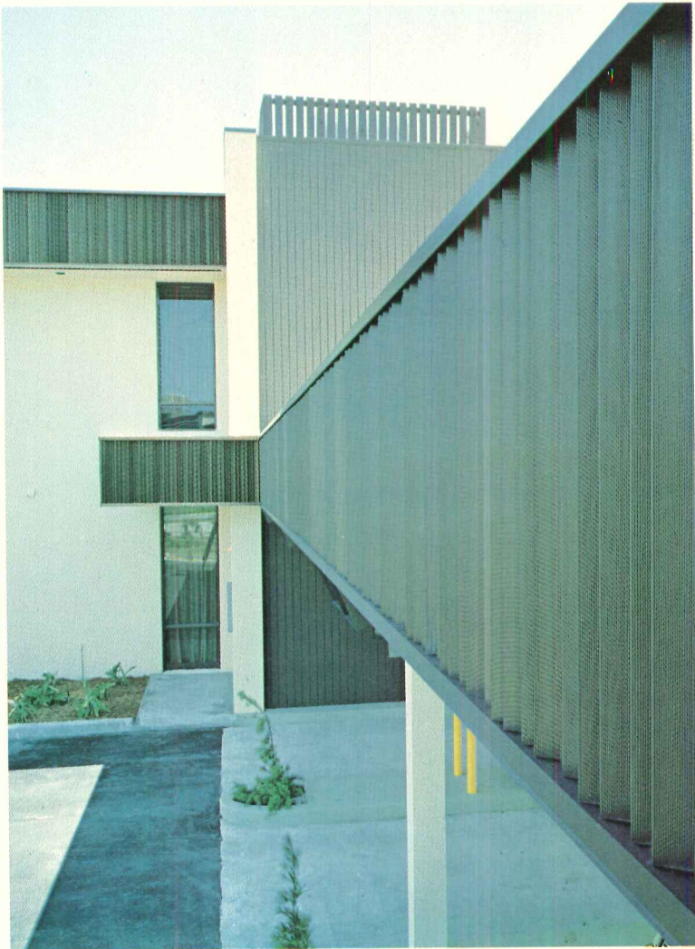
Project: Guardian Bank, Pinellas Park, Florida Architect: Robert Bernzott Fabricator: J-C Products Corporation Applicator: Midway Glass Company
