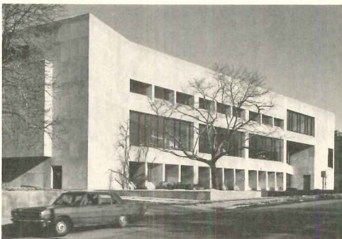
Waterbury (Connecticut) Courthouse, by Joseph Stein & Associates and Louis R. Fucito & Associates.
