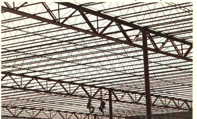
717 tons of joists and 433 tons of joist girders were used in this 746,852 square foot job.
