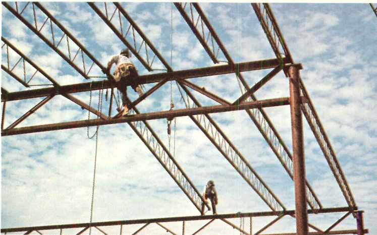
The simplicity and light weight of Vulcraft joists and joist girders make erection fast and easy.
