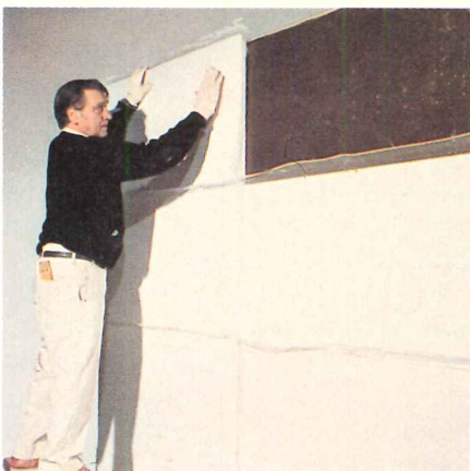
A plasterer demonstrates the ease and simplicity of the Thermoclad system, applied here over an 8 x 8 foot panel of exterior gypsum over metal studding. In the first photo, Thermoclad insulation,
