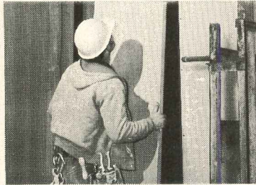
2. Installing core panel.
