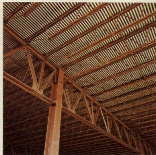
Joist girders have top chord panel points that show joist location. Which makes a lot of measuring unnecessary.
