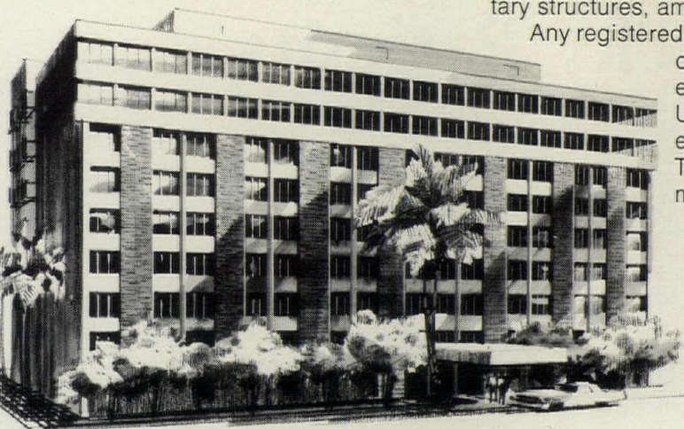
Boca Raton Community Hospital, Boca Raton, Florida.
