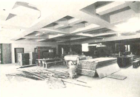
Photo above shows how a basic ceiling pattern can remain exposed in sections where mechanical and electrical requirements and interior finishes do not call for a suspended ceiling.
