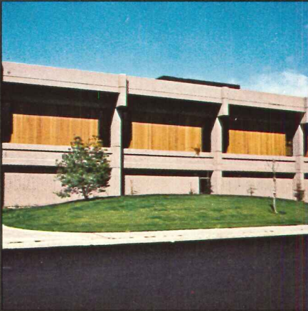
Ruf-Sawn redwood plywood combined with architectural concrete
