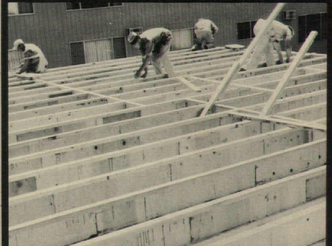
I Series joists go in place 2 to 4 times faster than 2 x 10's.
