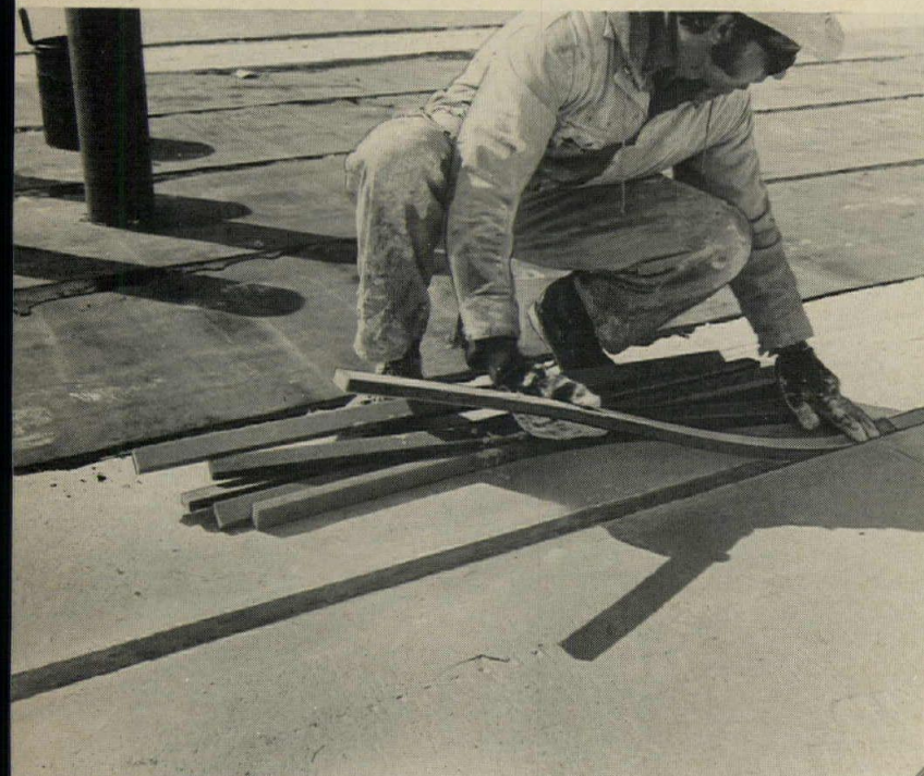
3 Precut polyurethane joint strips provide uniform insulation factor for entire deck.
