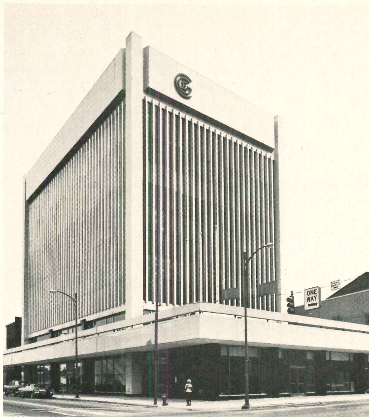
The Cincinnati Gas and Electric Company's Northern Division Offices, Middletown, Ohio. Architects: Gartner, Burdick, Bauer-Nilsen, Cincinnati, Ohio. Contractor: Frank Messer and Sons Construction Co., Cincinnati, Ohio.
