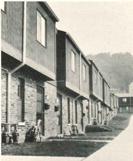
The Project: Westgate Village, 230 Units, Crafton-Ingram Section, Pittsburgh, Penna. Contractor/Builder: Mellon Stuart Company, Pittsburgh, Penna.
