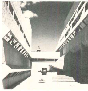
Cover: Physical Sciences Complex, University of Guelph, Guelph, Ontario Architects: Craig, Zeidler & Strong Photographer: Michel Proulx
