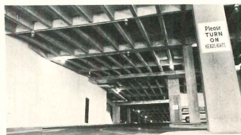
Large, open parking ramps. Lightweight concrete in long-span floor joists gave lowest possible weight for required fire rating without ceilings.
