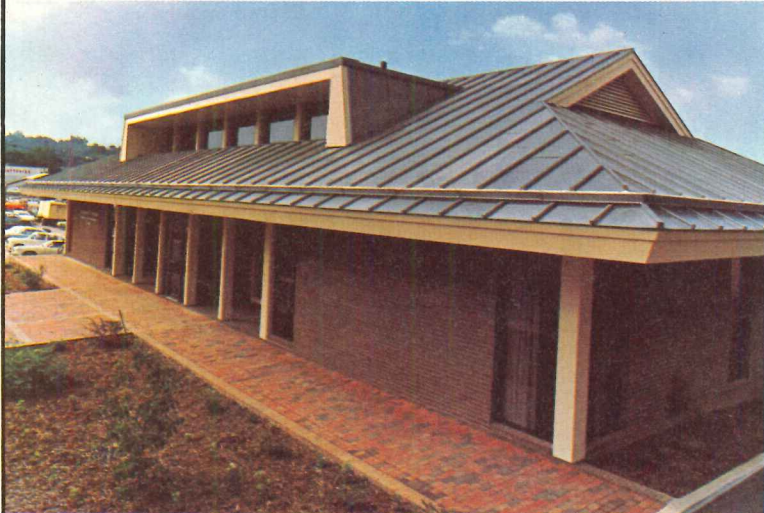
GREENEVILLE FEDERAL SAVINGS & LOAN • GREENEVILLE, TENNESSEE Architect: Boyd & Arthur • Roofing & Sheet Metal: Hicks Sheet Metal Co.
