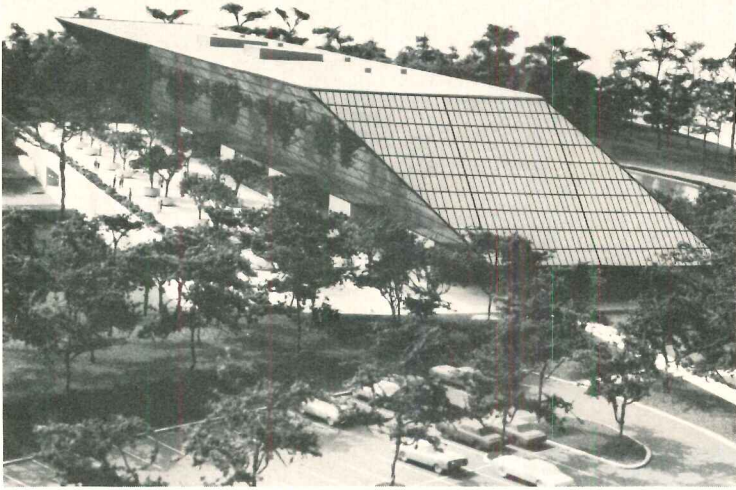
The North Carolina Blue Cross and Blue Shield Headquarters Building , by architects Odell Associates Inc., displays a new shape for reflective glass buildings—a 500-foot-long, 100-foot-wide rhomboid. Now being constructed on a 39-acre tract
