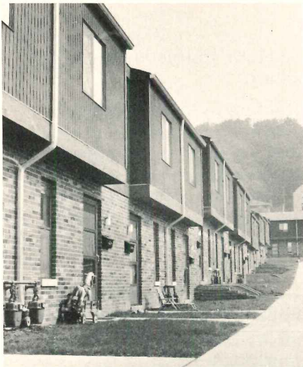
The Project: Westgate Village, 230 Units, Crafton-Ingram Section, Pittsburgh, Penna. Contractor/Builder: Mellon Stuart Company, Pittsburgh, Penna.
