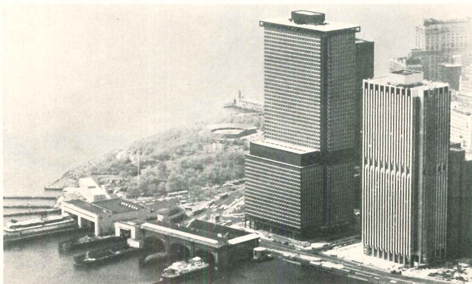
2 New York Plaza (at right in the adjoining photo) completes the third and final building in the New York Plaza complex at the southern tip of Manhattan. The entire complex was sponsored by the Sol G. Atlas and John P. McGrath investment partnership. Architects for this new 40-story tower are Kahn and Jacobs, with Nevio Maggiora as project designer. The building contains a total of 1,300,000 sq ft, including a shopping level (reached by a sunken plaza) beneath the building's five-foot podium. The aluminum-clad structure has a steel frame with 40-foot spans, crossed-braced steel center core.
